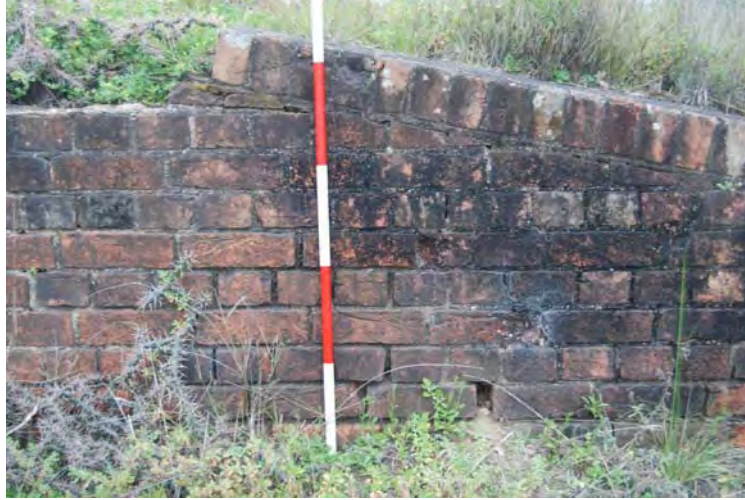
Photo: DSC_0176; View: west
