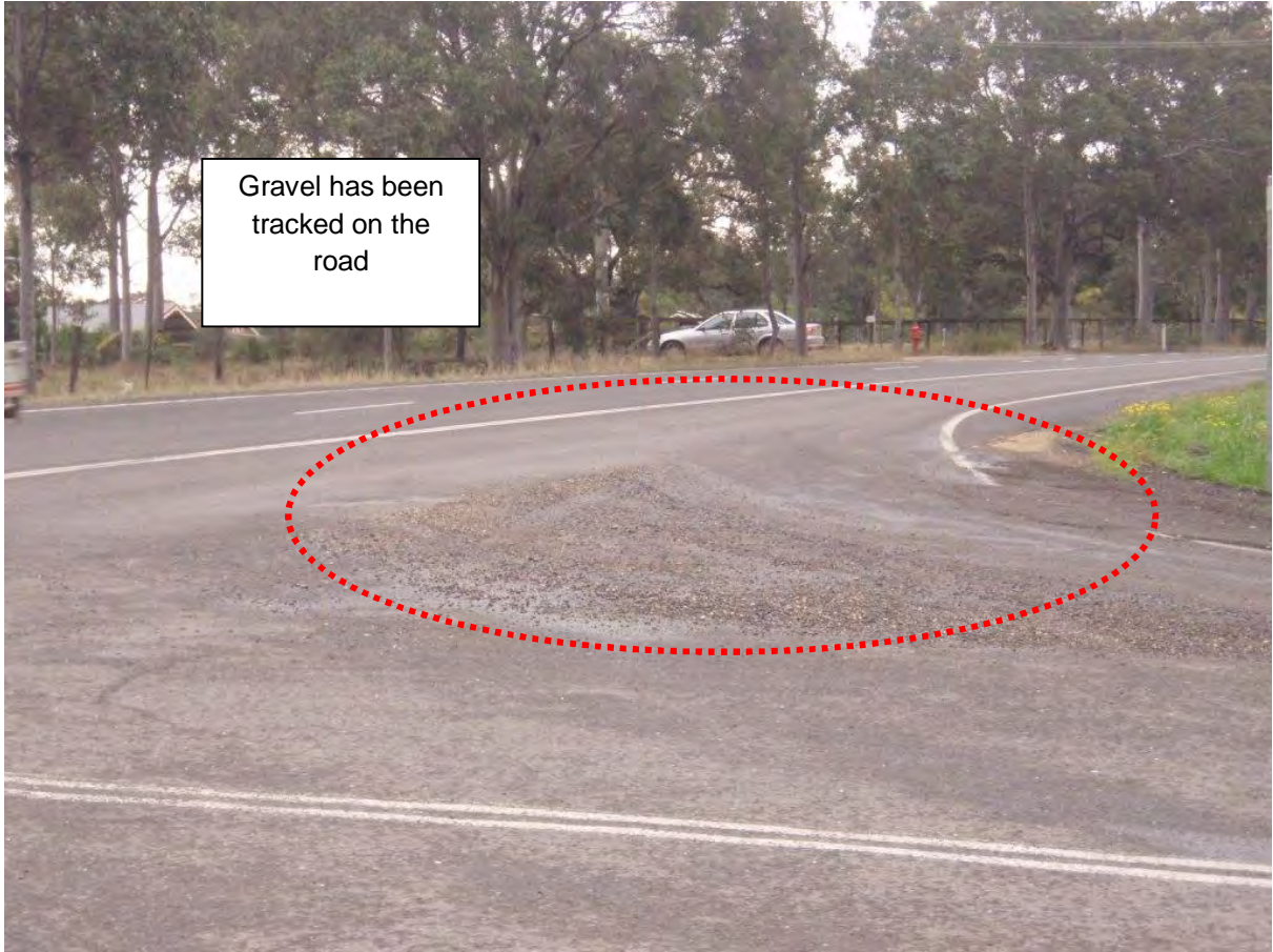
Photo 11 Looking north from Retreat Road towards Bridgman Road
