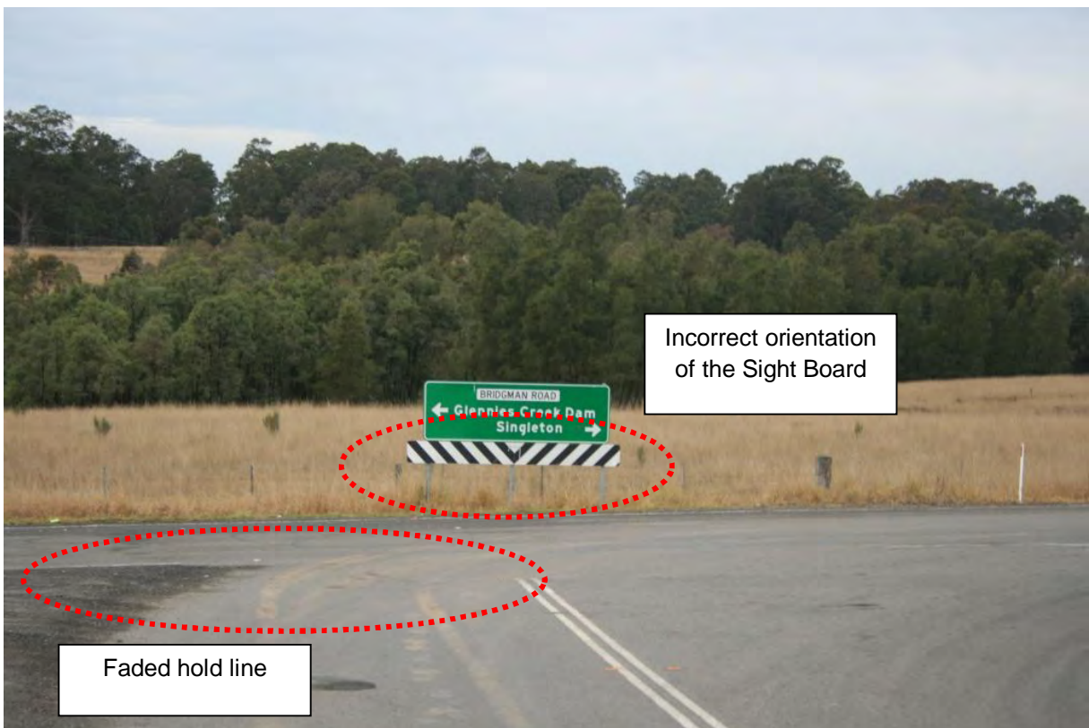
Photo 16 Stoney Creek Road on approach to its intersection with Bridgman Road
