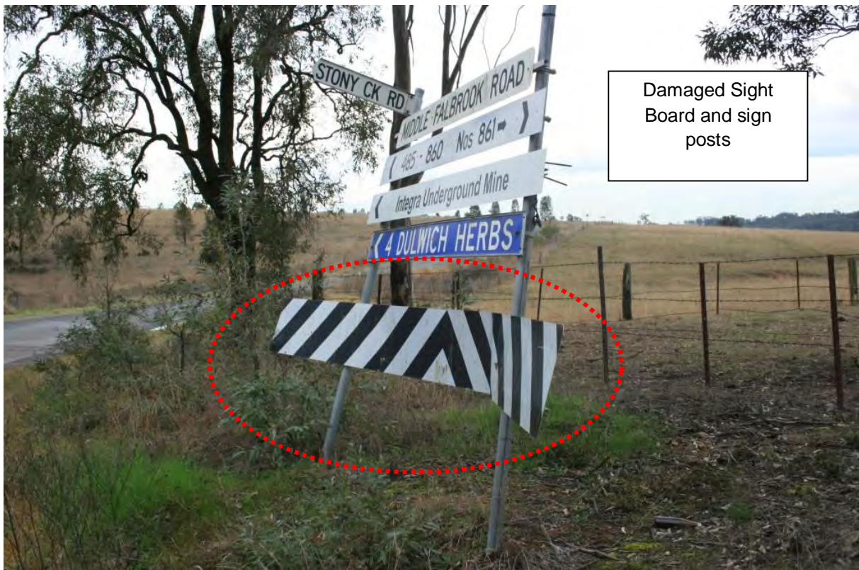
Photo 18 Middle Falbrook Road/ Stoney Creek Road intersection
