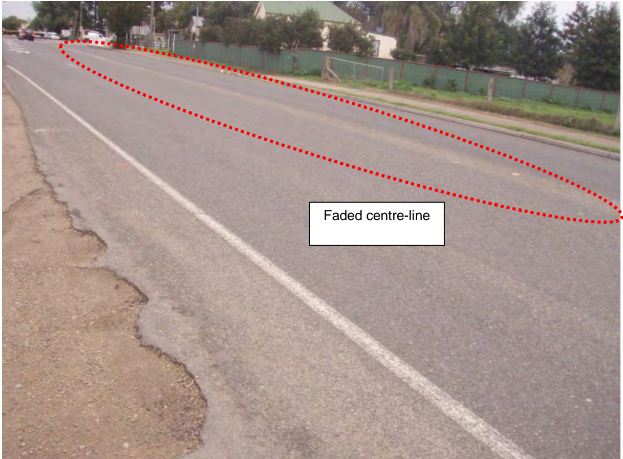
Photo 7 Bridgman Road, looking south towards its intersection with New England Highway
