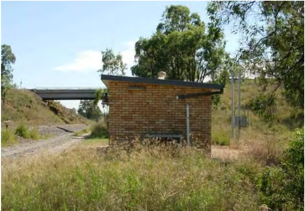
Photo 8.1a Camberwell Relay Room
