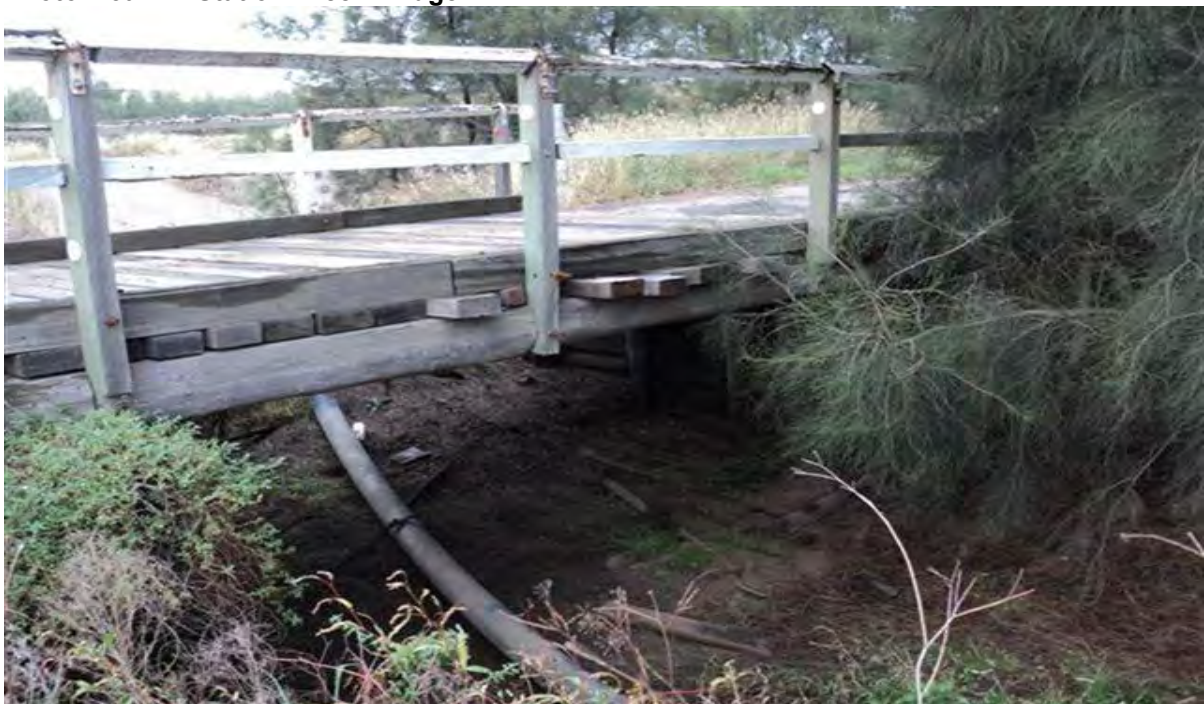
Photo 4.3a Station Creek Bridge
