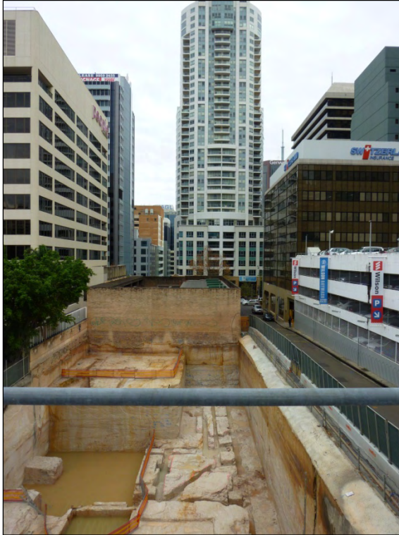
Figure 9-38 – View of the Proposed Substation and Existing Substation Sites in the Foreground Surrounded by North Sydney Development Looking South
