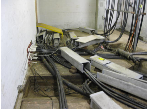
Plate 1: Asbestos cement cable troughs to South west cable room
