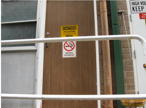
Plate 13: White lead paint to door frame of lunch room
