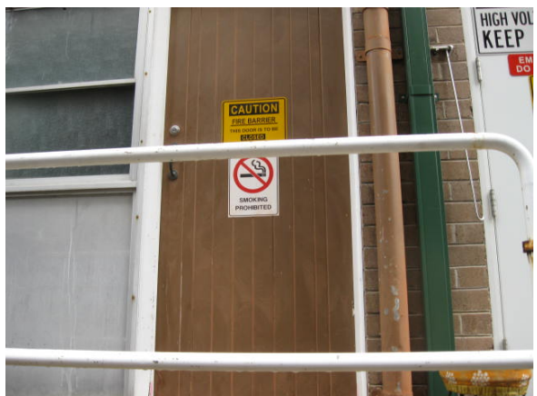
Plate 12: Lead paint to external brown paint to electrical conduits and pipes.
