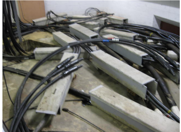
Plate 2: Asbestos cement cable troughs to North West cable room
