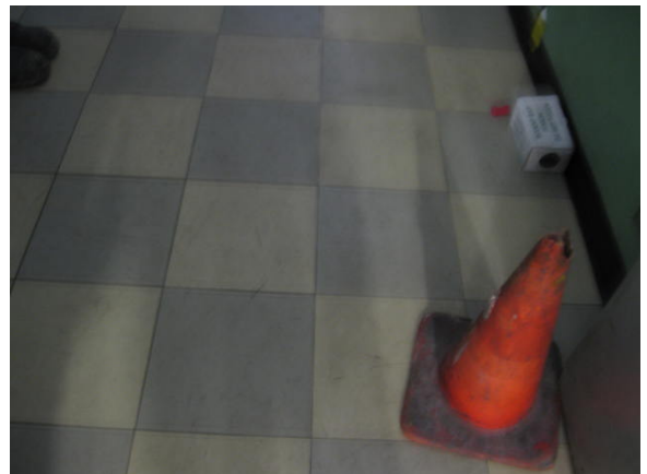
Plate 4: Vinyl floor tiles to Battery room sampled and found not to contain asbestos after laboratory analysis.
