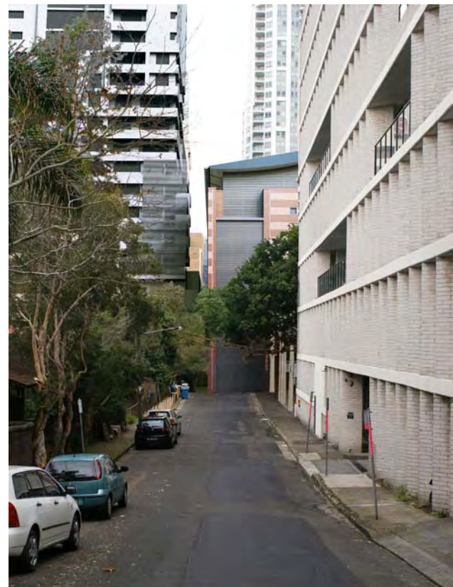
Figure 3.5.1: Photomontage of view down Harnett Street from McLaren Street with proposed substation and proposed residential development at 136-140 Walker Street (Source: Kann Finch Group)
