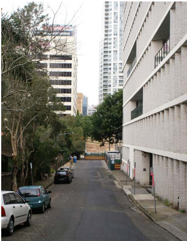
Figure 3.2.1: View down Harnett Street from McLaren Street
