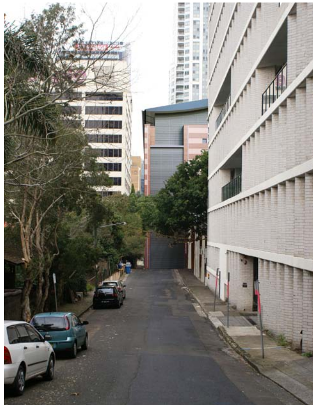
Figure 3.2.2: Photomontage of view down Harnett Street from McLaren Street with proposed substation (Source: Kann Finch Group)
