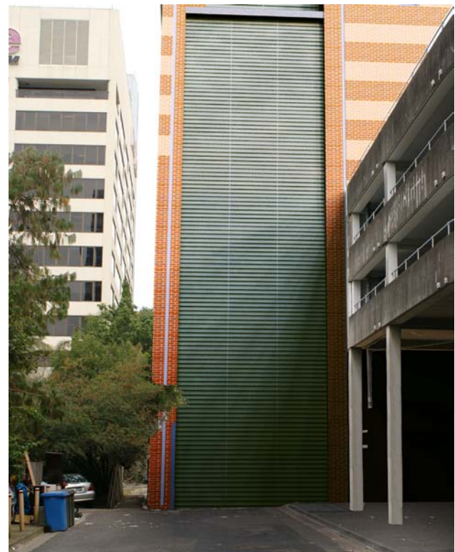
Figure 3.3.2: Photomontage of view middle of Harnett Street (Source: Kann Finch Group). The lower portion of the horizontal banded metal area is a roller door, the upper portion are louvres for ventilation.
