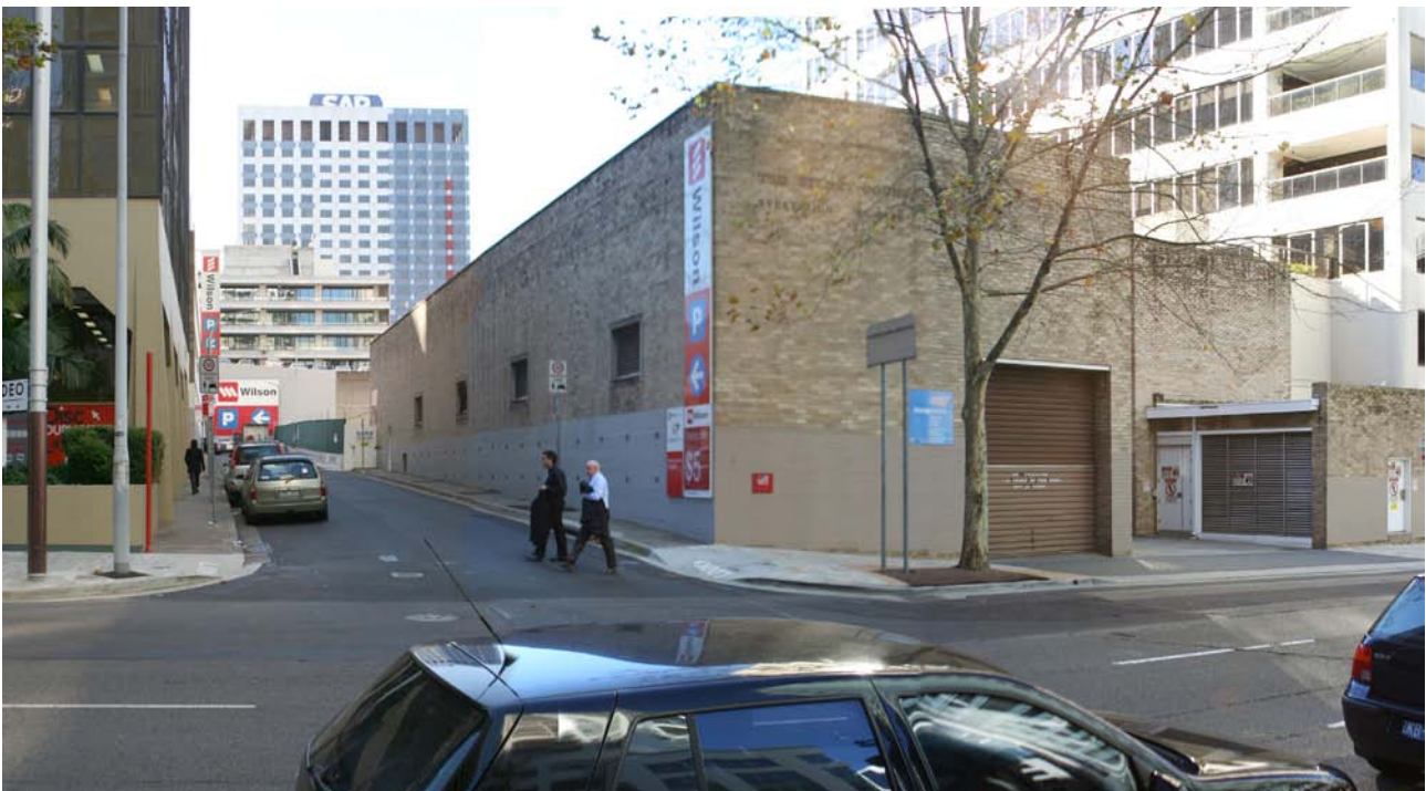
Figure 3.1.5: Panorama of Berry Street showing existing substation
