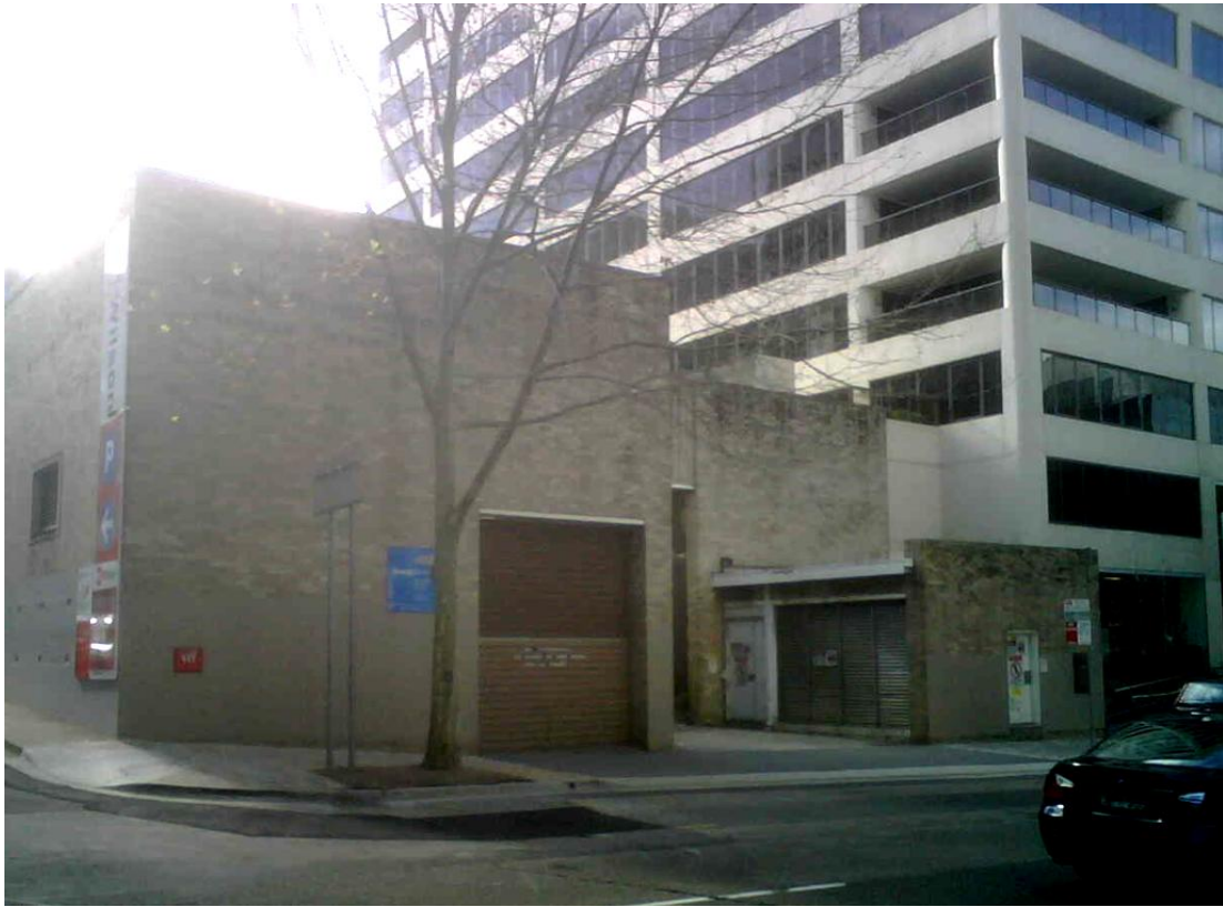
Figure 6-2 – Southern boundary (view of existing substation)
