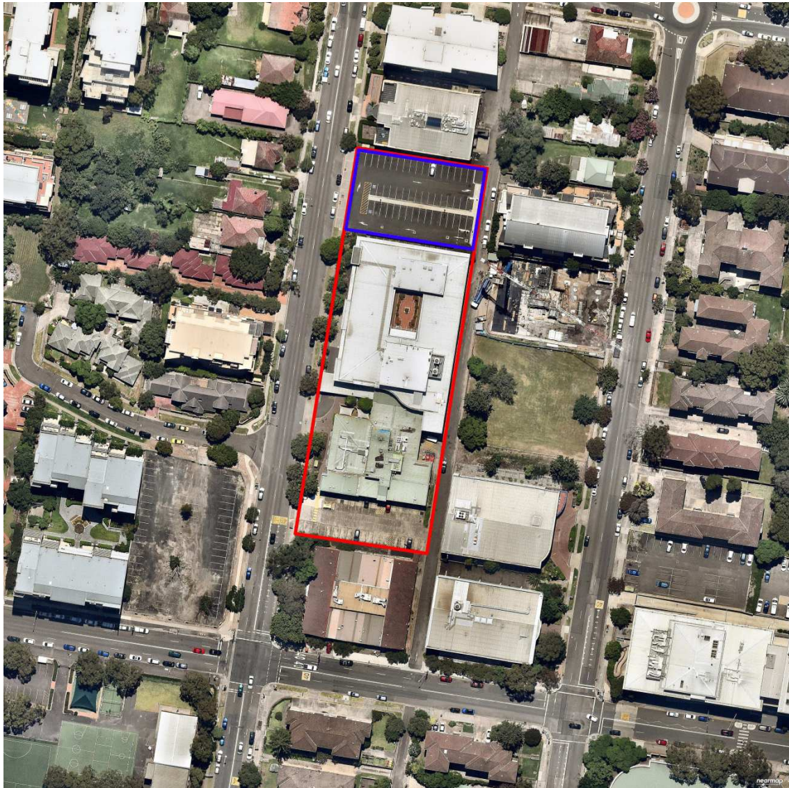
Figure 2 – Aerial photo, showing the existing hospital (red) and extension development site (blue). Source: Nearnmap
