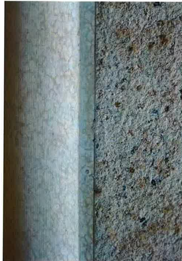
PRECAST CONCRETE FACADE (WD:01)
