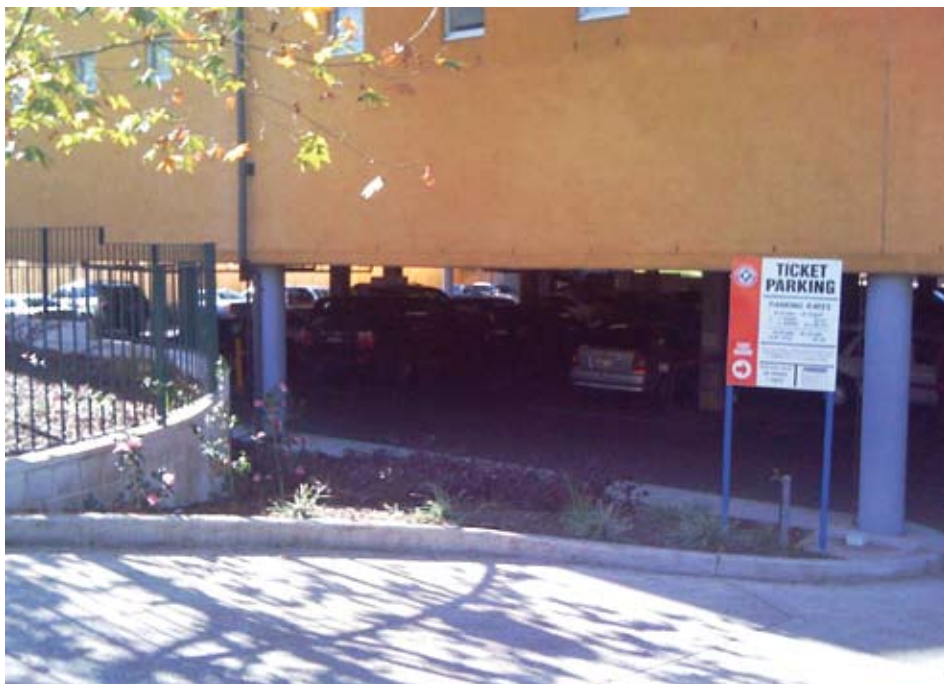
Figure 4 – Existing entrance to partially underground car park.
