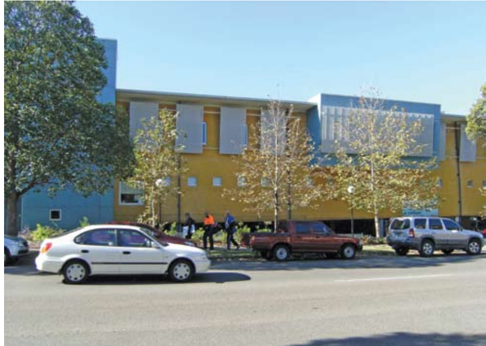
Figure 3 – Western facade of the existing hospital building.
