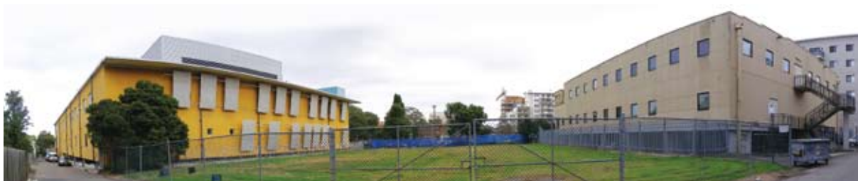
Figure 5 – Vacant northern portion of site.
