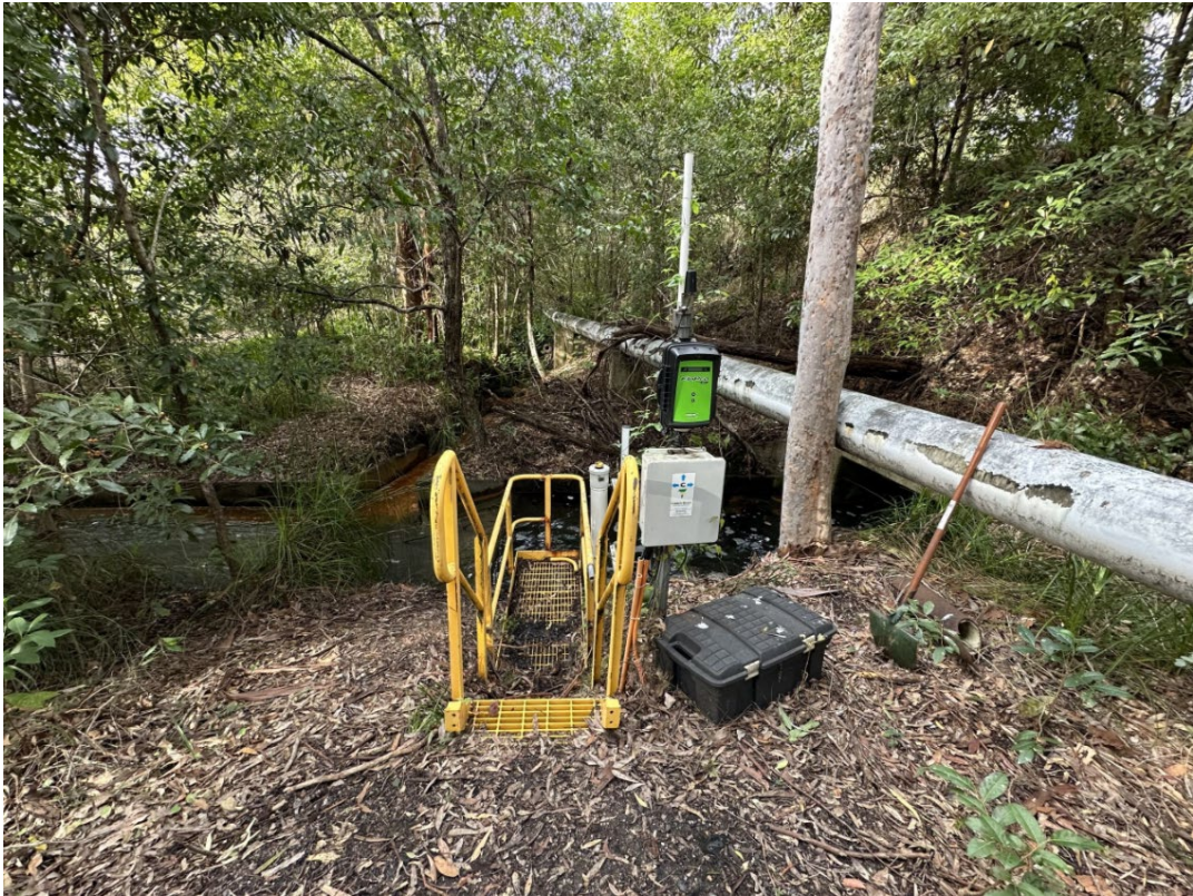
Photograph 41 – Licenced Discharge Point 9.
