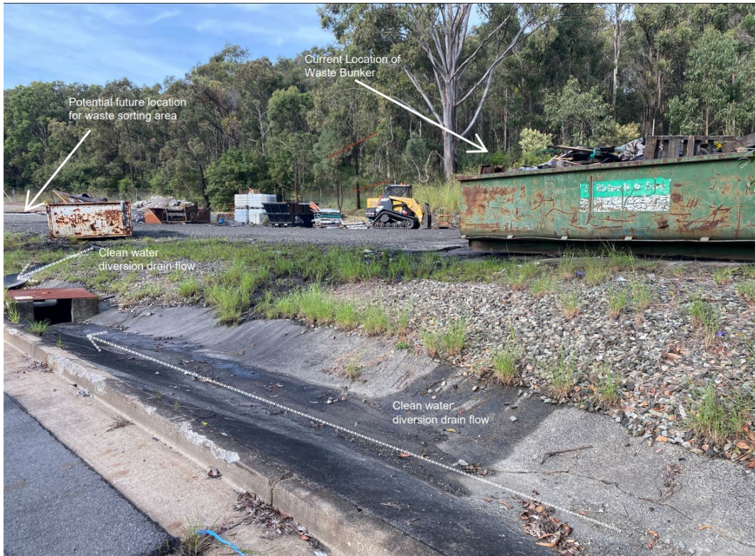
Photograph 31 – Waste sorting area with IEMA recommendation of potential future location for waste sorting area.
