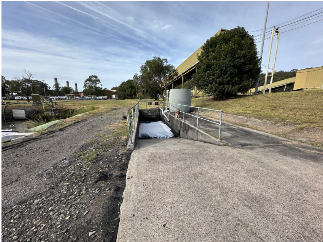
Photograph 34 – Primary Settlement Tank.
