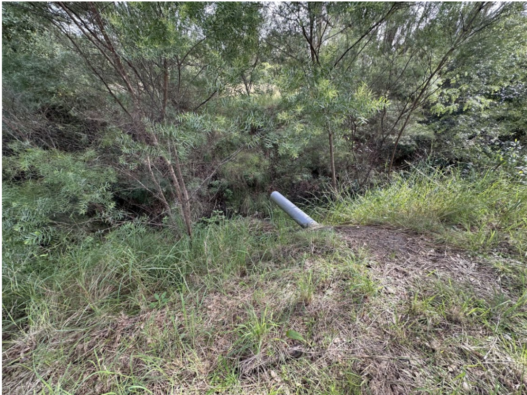
Photograph 46 – Licenced Discharge Point 10.
