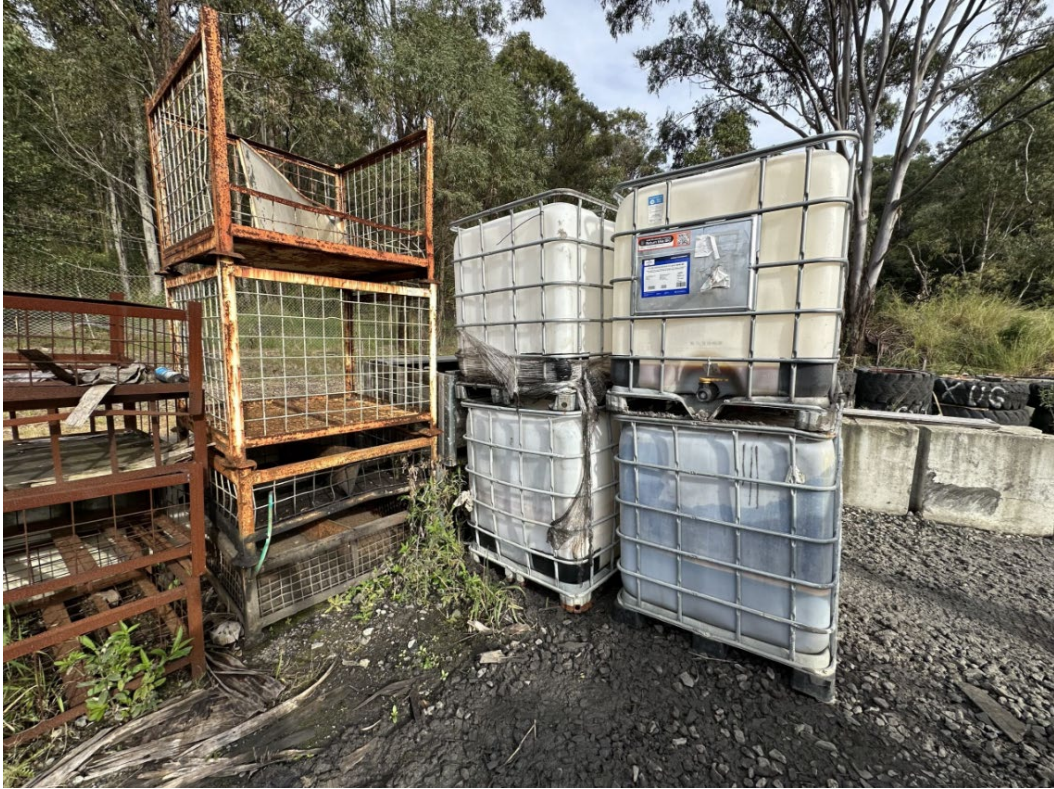
Photograph 23 – Hydrocarbons incorrectly stored (not banded) adjacent to waste sorting area. Does not meet AS1940.
