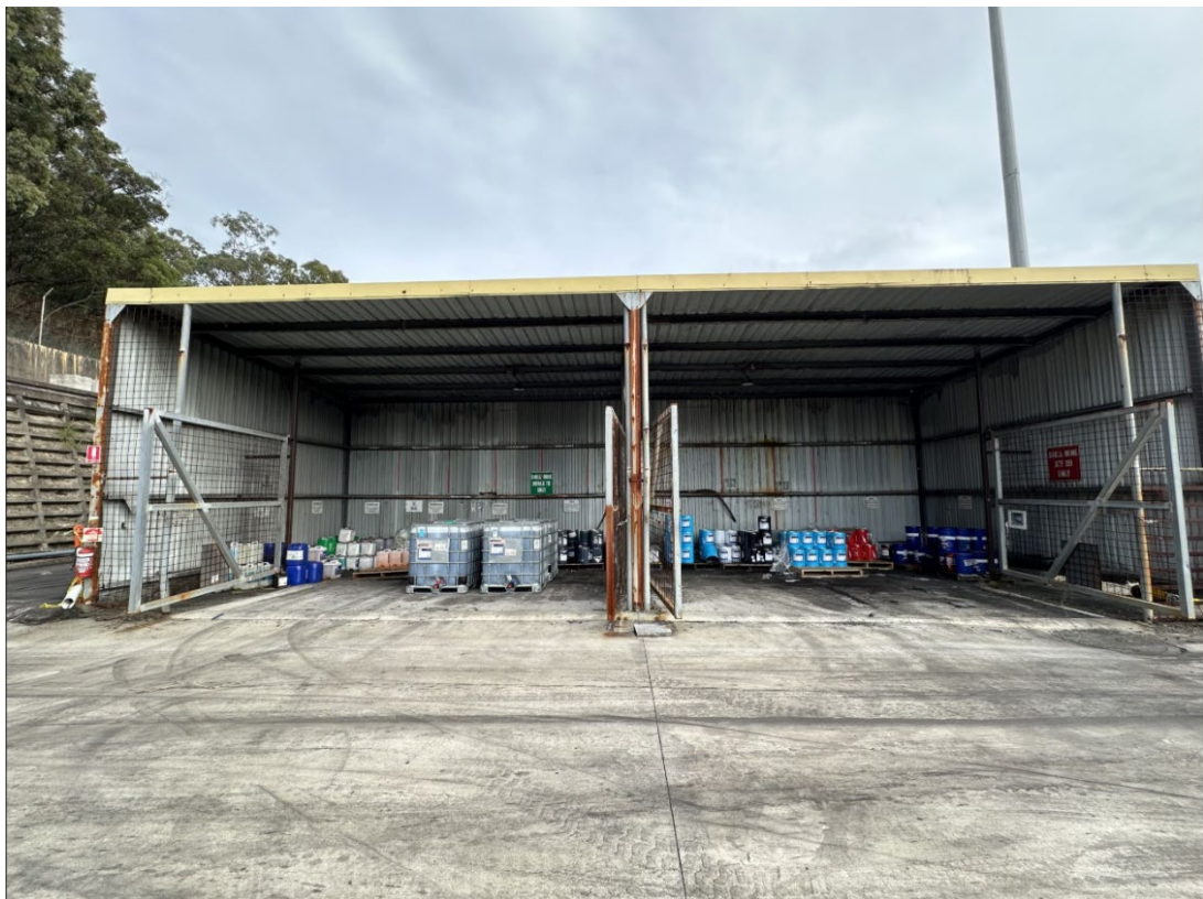
Photograph 10 – Bunded hydrocarbon storage shed.
