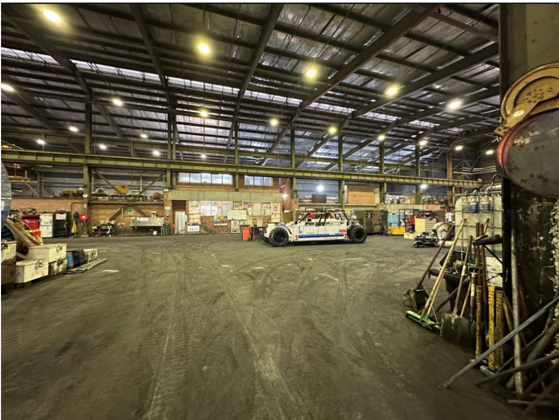
Photograph 06 – Inside of Workshop.
