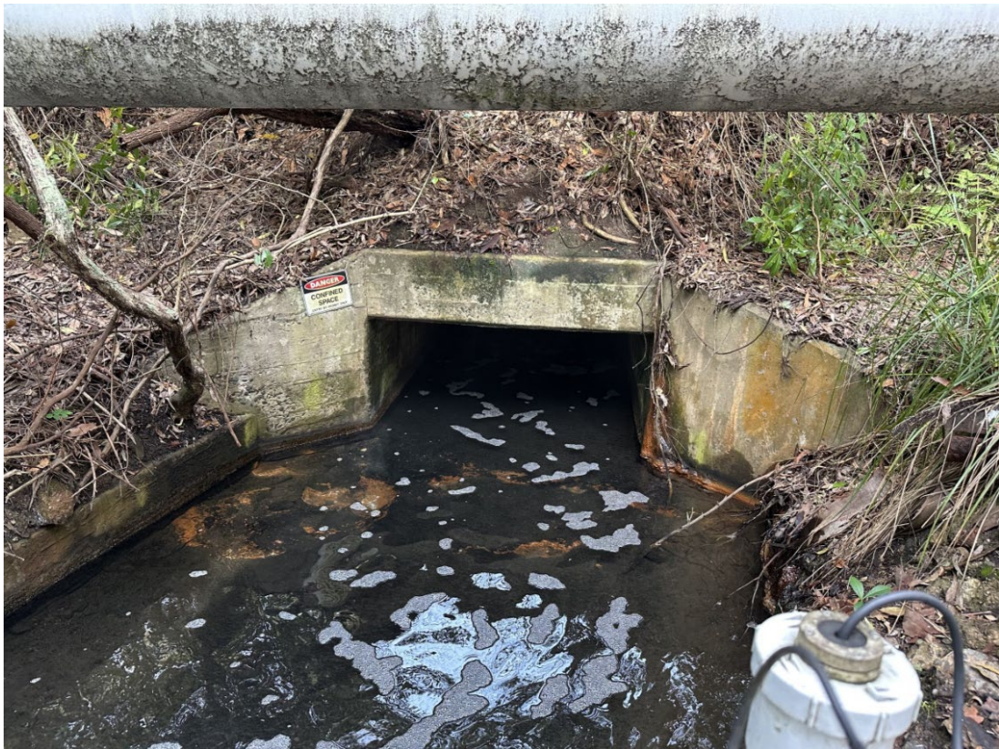
Photograph 40 – Licenced Discharge Point 9.
