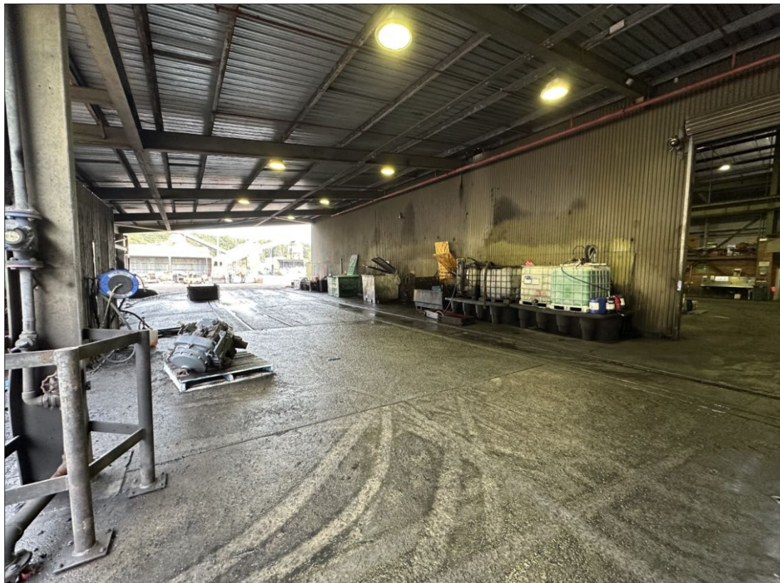
Photograph 08 – Hydrocarbon storage in Workshop Washdown Bay.
