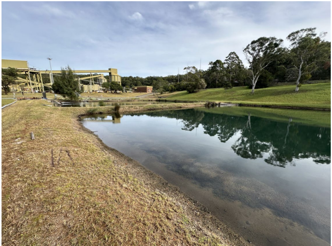
Photograph 36 – Mine Water Settling Ponds 2 and 3.
