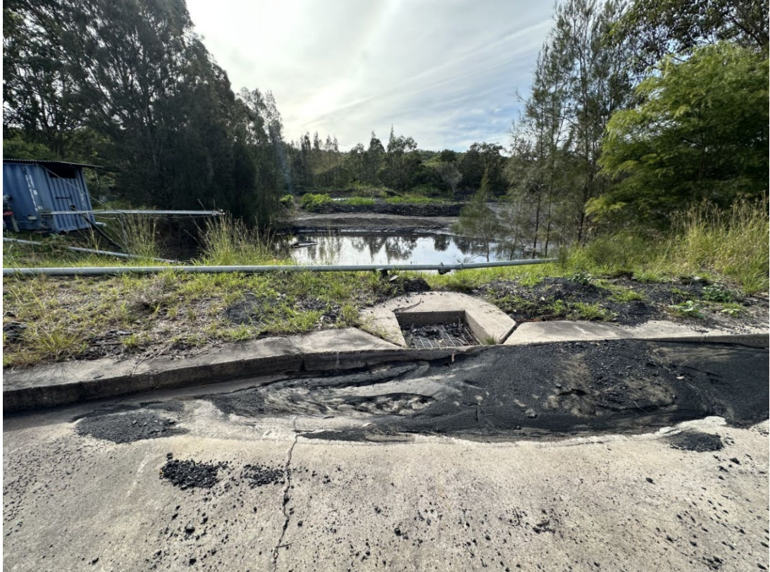
Photograph 45 – Emergency Coal Stockpile Dam.
