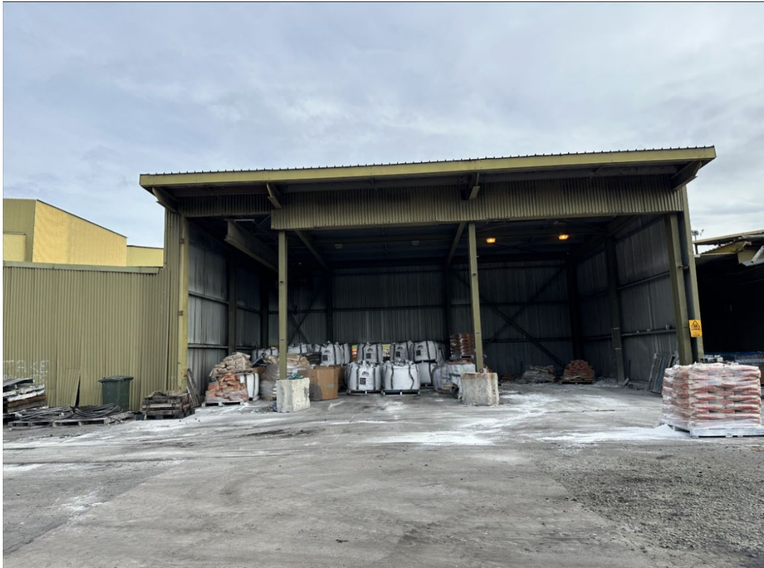
Photograph 13 – Stone dust storage shed.
