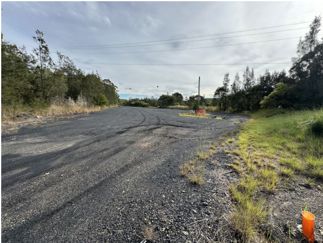
Photograph 44 – Emergency Coal Stockpile Area.
