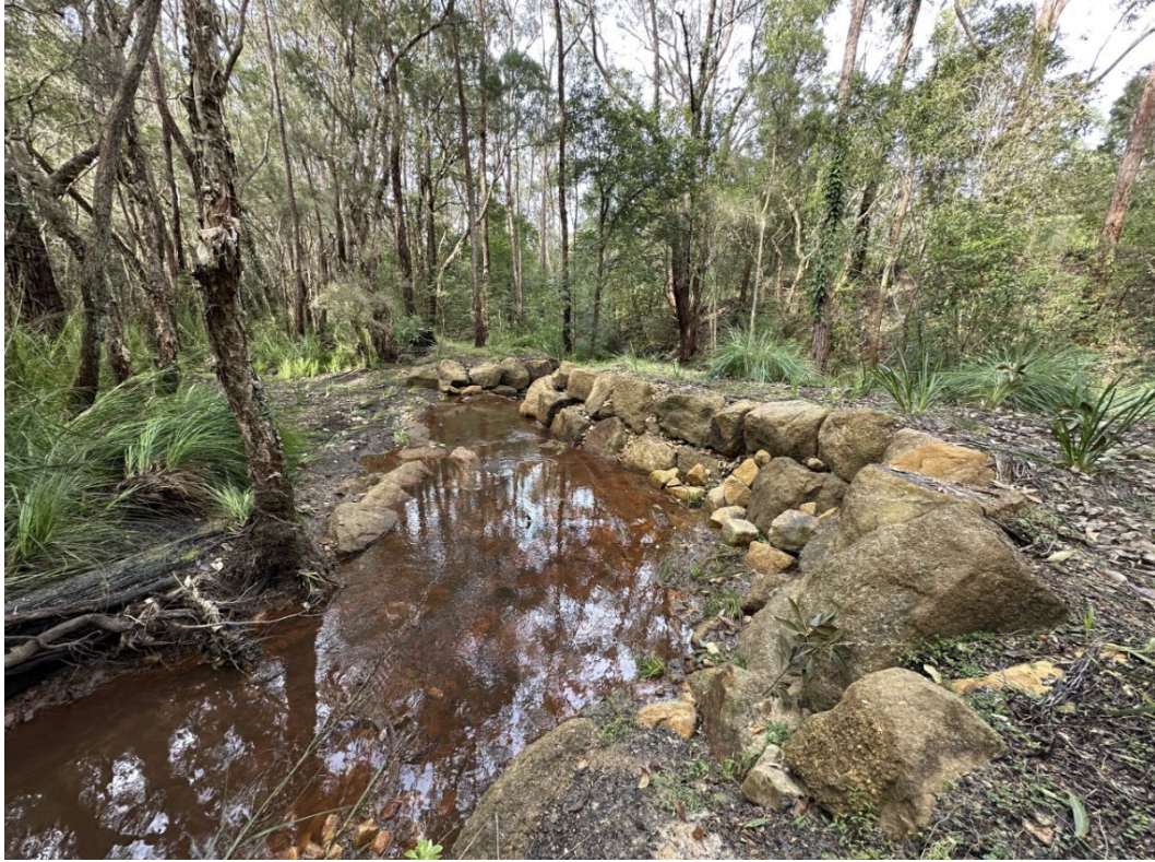
Photograph 43 – Wangi Creek remediation works.
