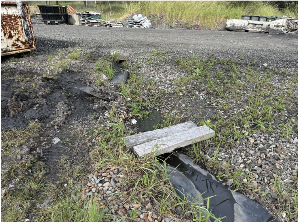
Photograph 28 – Clean water diversion drain running under the waste sorting area.
