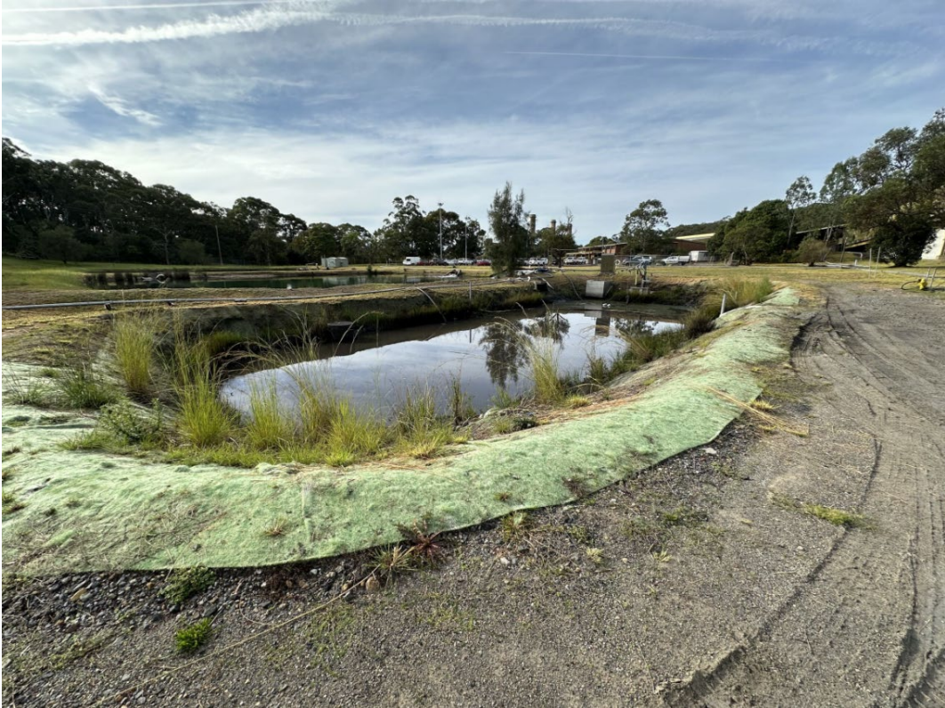
Photograph 33 – CHP Dam (Mine Water Settling Pond 1).
