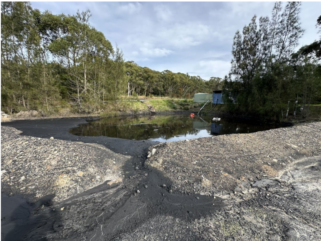
Photograph 48 – Emergency Coal Stockpile Dam.
