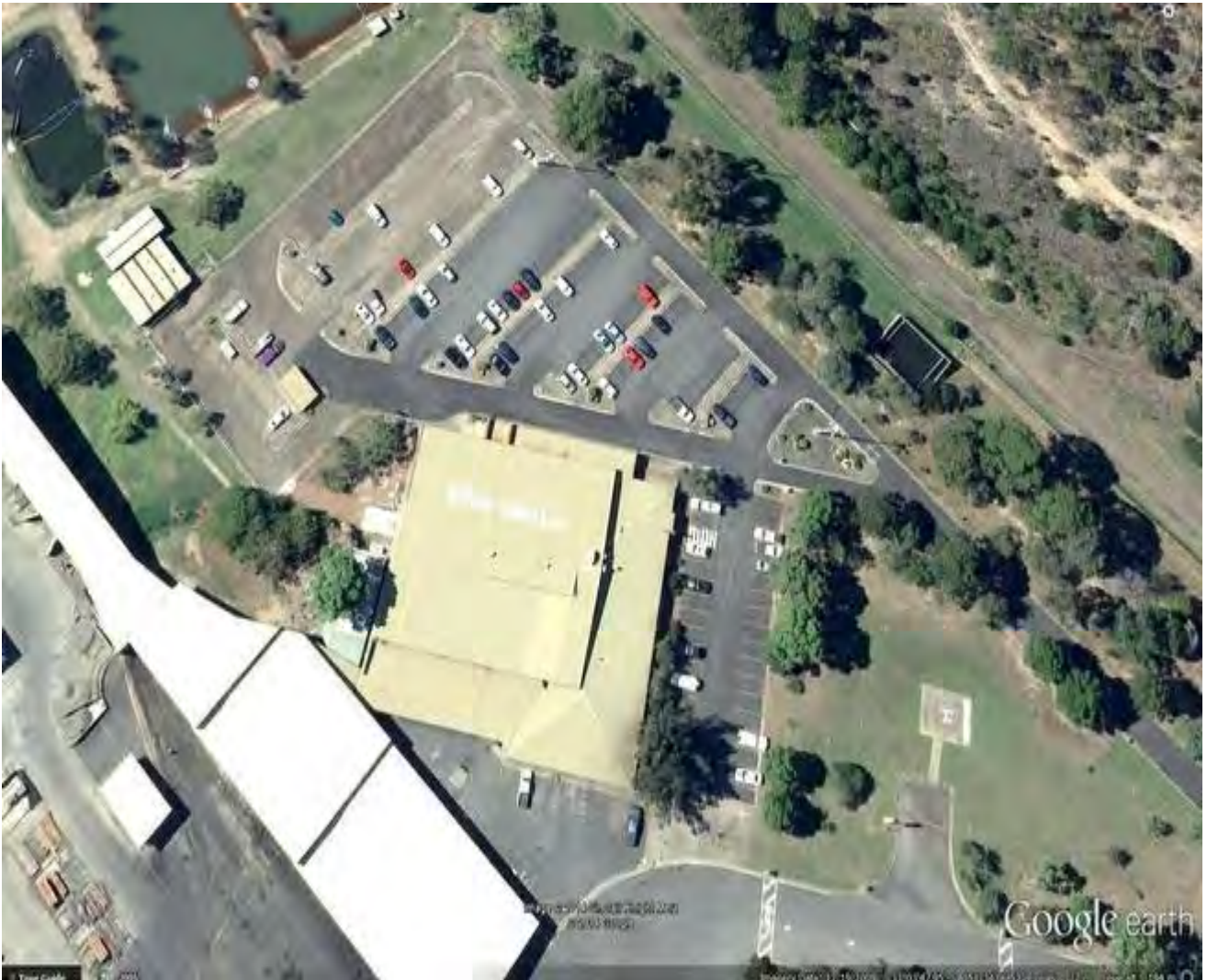
Figure 5 – Existing Myuna Colliery car parking areas
