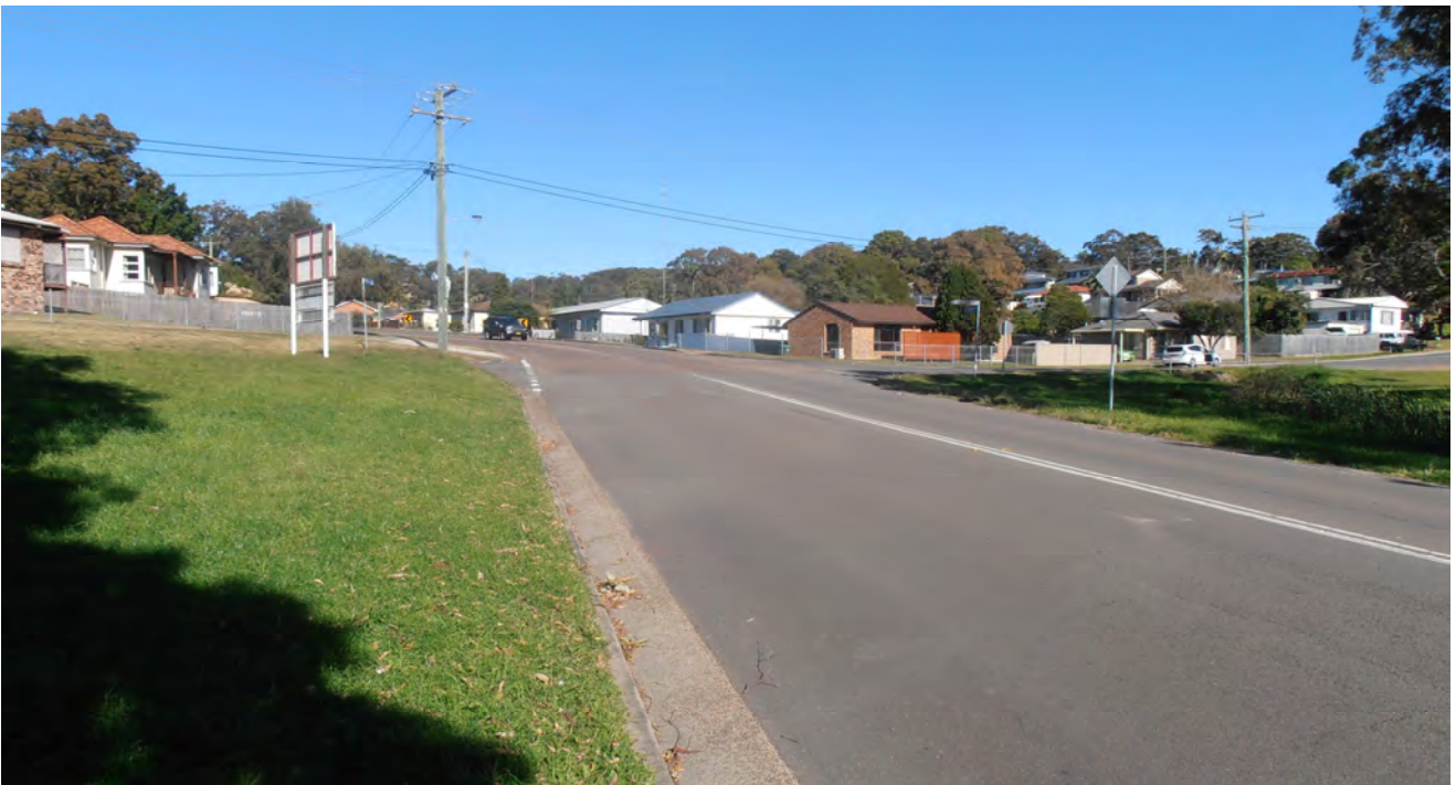
Photograph 3– Donnelly Road in the vicinity of Dobell Drive
