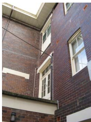
Figures 3.16 and 3.17 (left and right) Timber framed doors and windows in the east and south facades that could be salvaged
