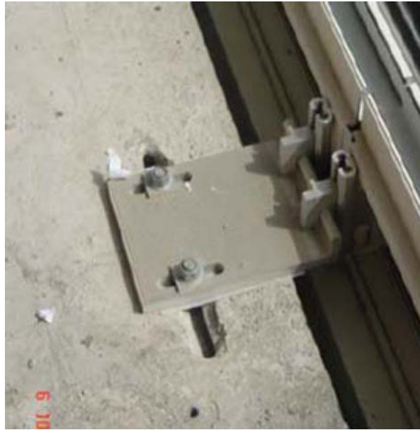
Figure 7 : Curtain wall bracket (top of slab fixing)
