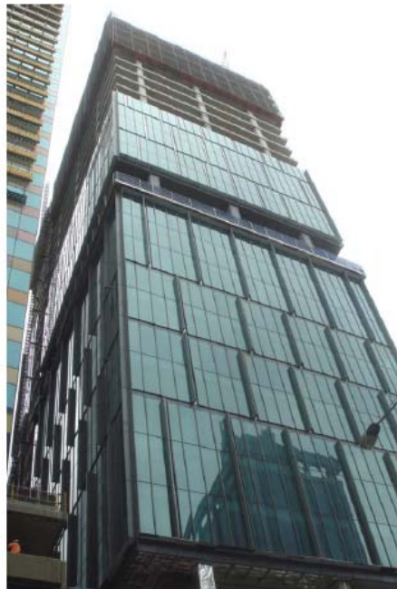
Figure 1 : 400 George Street Brisbane, Curtain wall (during construction)
