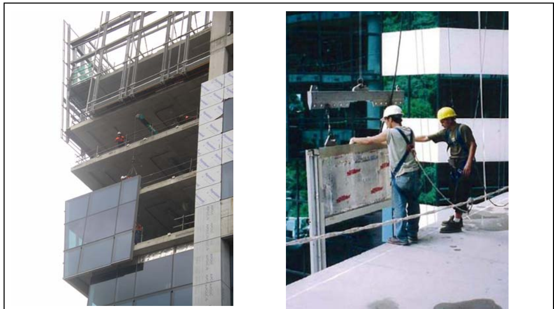
Figure 9 : Installation of unitized curtain wall
