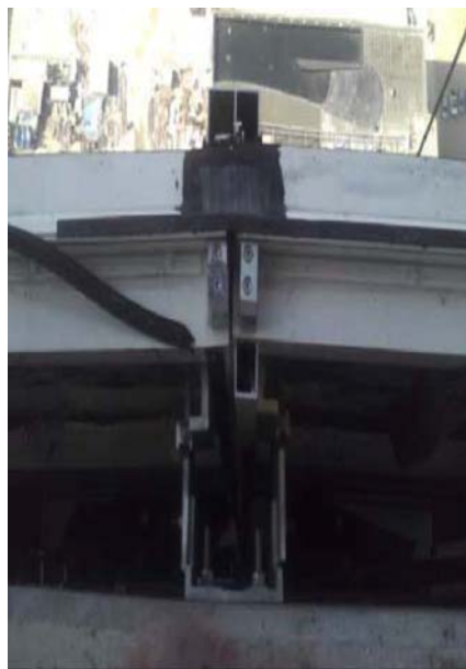
Figure 8 : Curtain wall bracket (slab face fixing)
