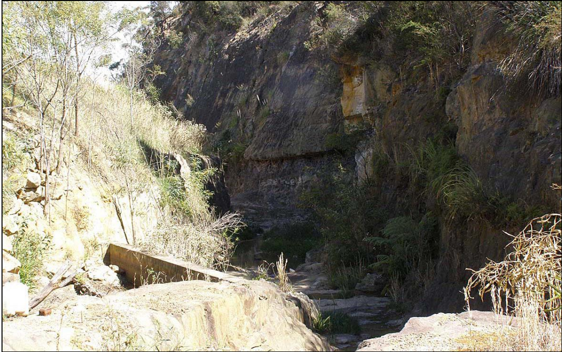
Plate 6.7 – Mechanically-excavated drainage channel along the western boundary.
