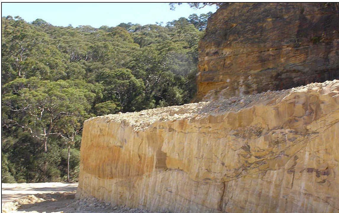
Plate 6.10 – Excavated benches in the north-western section.
