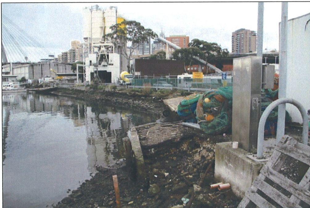
Figure 24: Existing Blackwattle Bay Foreshore at SFM
