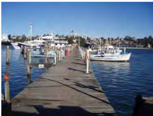
Wooden deck wharf servicing the Harbour Fleet
