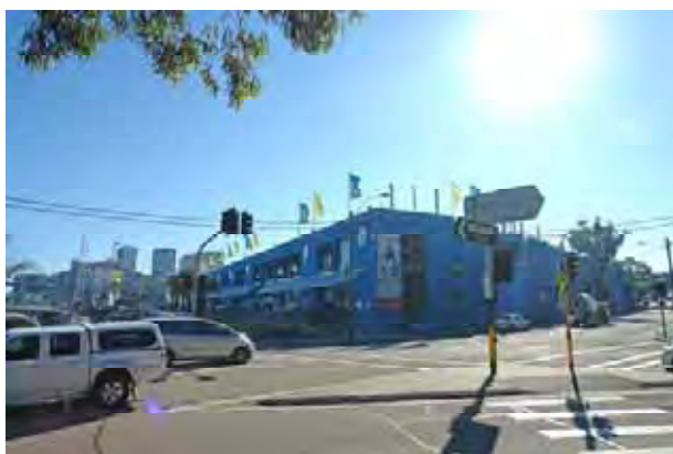
View from Pyrmont Bridge Road/ Wattle Street intersection
