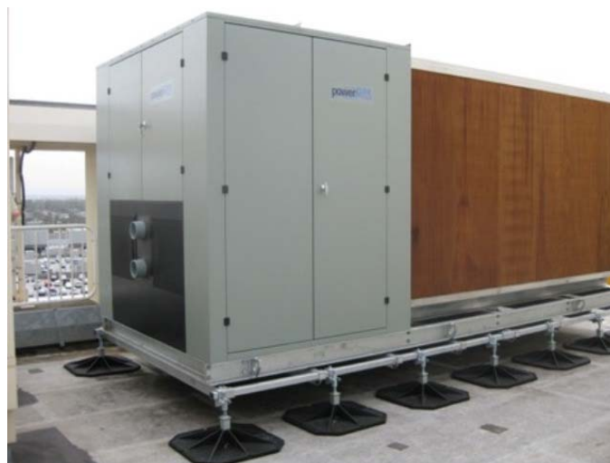
Typical Air cooled chiller installation.
