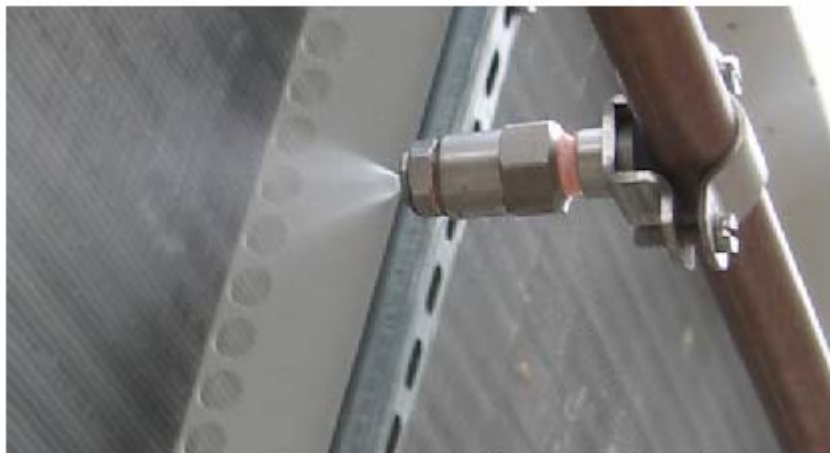
Typical Water Spray Nozzle Installation
