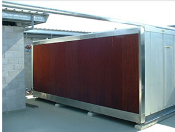
Typical Fluid Cooler Installation with wetted pads
