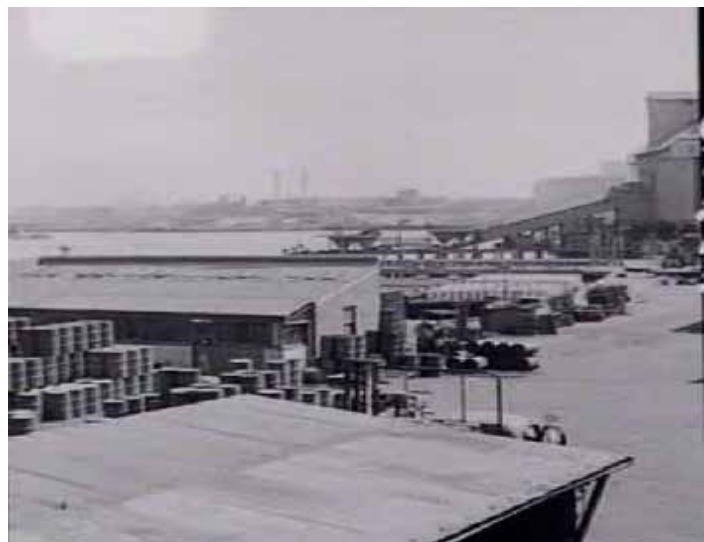
Three views of the Shell Oil Depot at the time it was taken over as the site for the new fish market (ML d2-30745, d230746, d2-30756)
