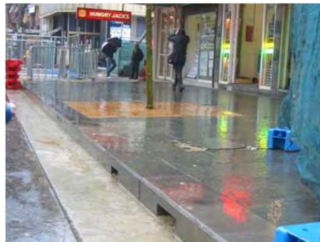
Kerb opening in Darlinghurst
