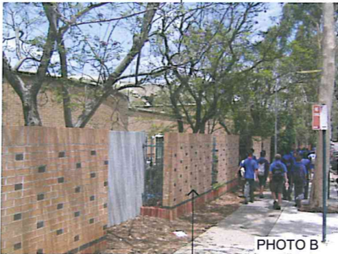
PART OF EXISTING BOUNDARY WALLS TO BE DEMOLISHED
