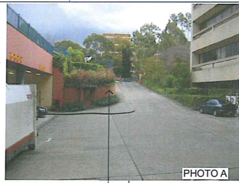
CARPARKING, RETAINING WALL, LANDSCAPING & METAL FENCING TO BE DEMOLISHED
