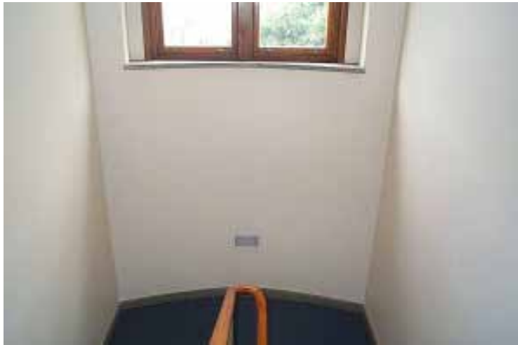
Figure C4: Image of the stair mid-landing. Note the curved wall and curved terrazzo window sill. OCP 2006
