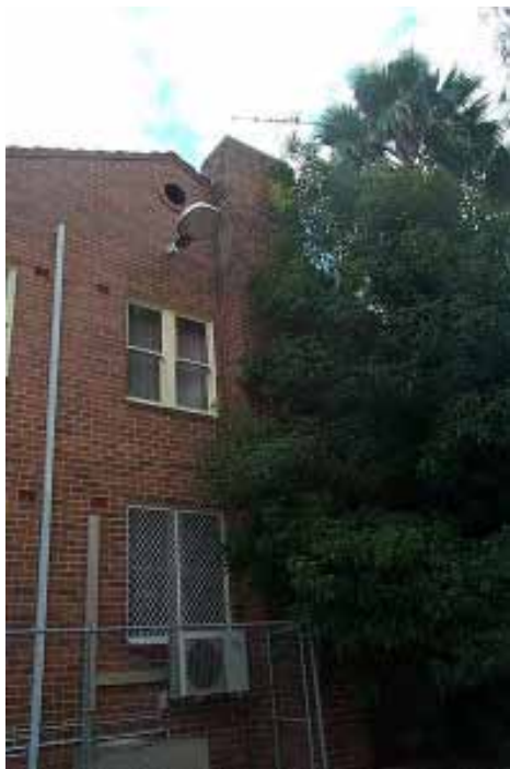
Figure C12: Image of the East Elevation with the chimney stack. OCP 2006
