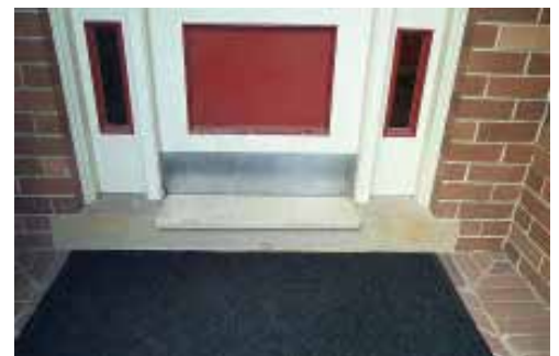
Figure C13: Image of the entry threshold. Note the addition of the terrazzo step into the sandstone block. OCP 2006
