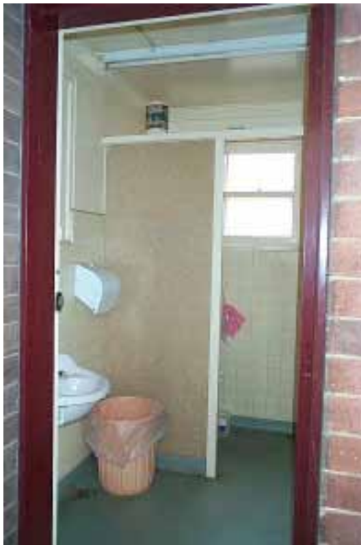
Figure D6: Image of a toilet with original tile and terrazzo finishes and fittings. OCP 2006
