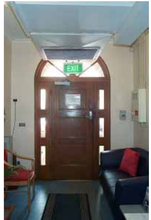
Figure C1: Image of the entry hall and front door. Note the air-conditioning duct. OCP 2006
