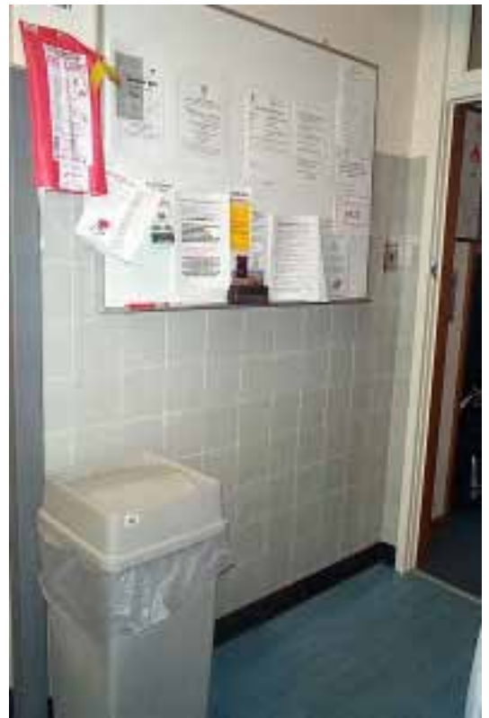
Figure C7: Original kitchen wall tile. OCP 2006
