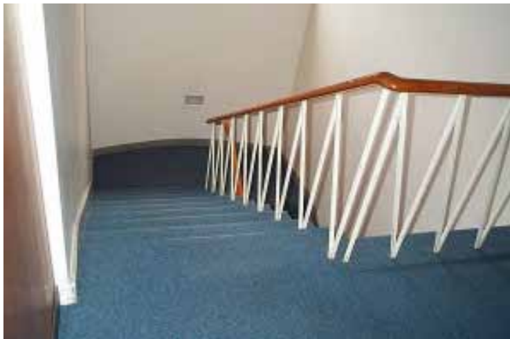
Figure C6: Image of the stairs from the first floor level. Note the timber handrail to the wrought iron balustrade. OCP 2006
