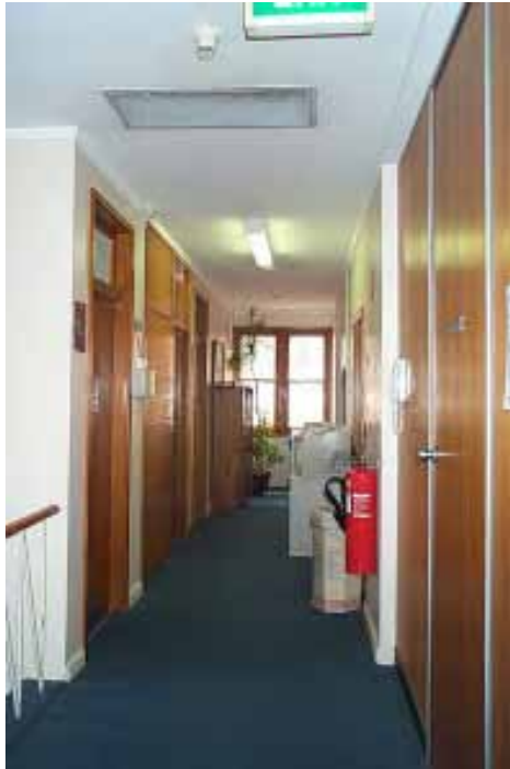
Figure C10: Image of the first floor hall, looking west. Note the timber finishes to the joinery and the double hung windows at the end of the hall. OCP 2006
