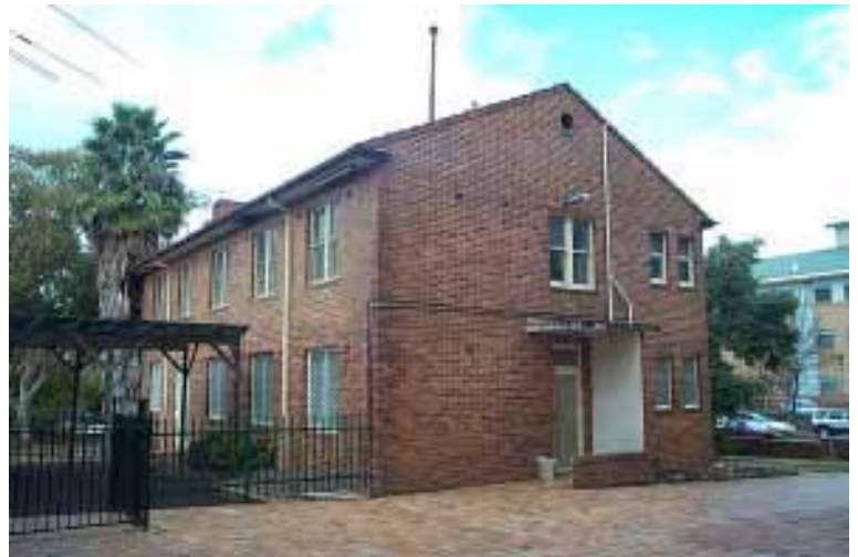
Figure C9: Image from the north west Note the side door entry canopy and the circular gable vent. OCP 2006
