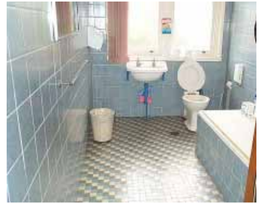
Figure 9: Image of the first floor bathroom at 1 Campbell Street. Note the original tiles and fittings. OCP 2006
