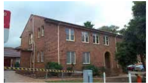
Figure 5: Image of I Campbell Street from the south west. OCP 2006
