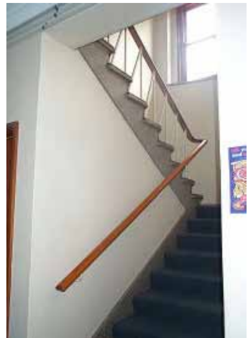
Figure 12: Image of the stairwell at 1 Campbell Street, from the ground floor. Note the terrazzo stringer and treads, as well as the wrought iron balustrade. OCP 2006
