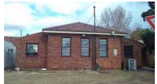
Figure 7: Image of the Hugh Jardine building from the north. Note the corbelled eaves and the horizontal glazing bars to the windows. OCP 2006
