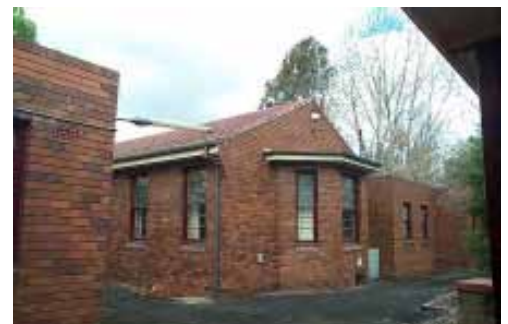
Figure 8: Image of the Hugh Jardine building from the west. Note the corbelled gable eaves, the bay window and the parapets. OCP 2006
