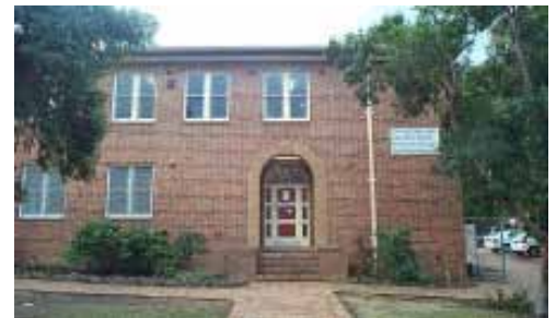
Figure 6: Image of I Campbell Street from the south. Note the sandstone arch to the entry portico. OCP 2006
