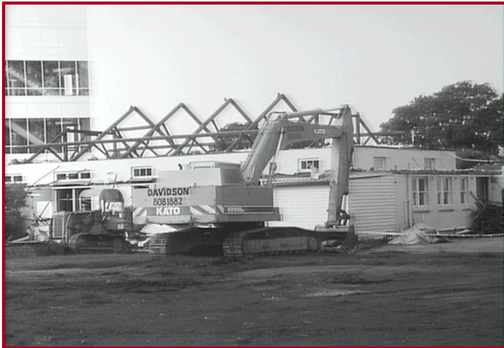
Figure 22. Demolition of “old” buildings, Liverpool Hospital site. (Picture 0672-16 Liverpool Library)
