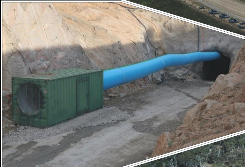
Plate 3: View of the Portal from western side of Box Cut with temporary fan and ventilation ducting
