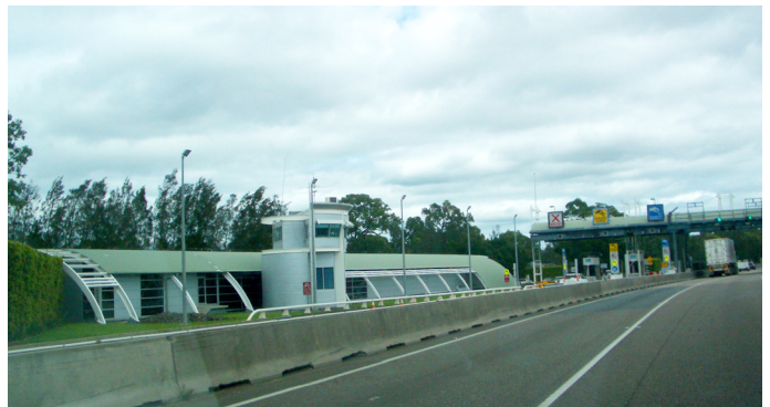
Illustration 11: The M5 control centre building at the toll plaza
