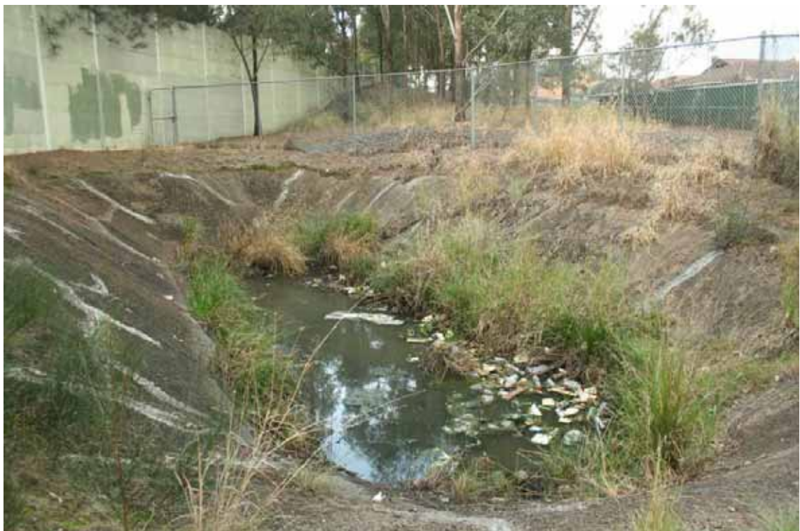
Plate 8: Concrete-lined sedimentation basin
