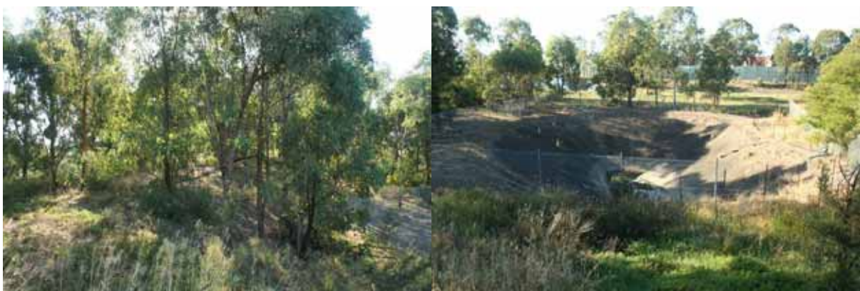
Plate 12: Planted vegetation on a fill batter (left), concrete detention basin (right)
