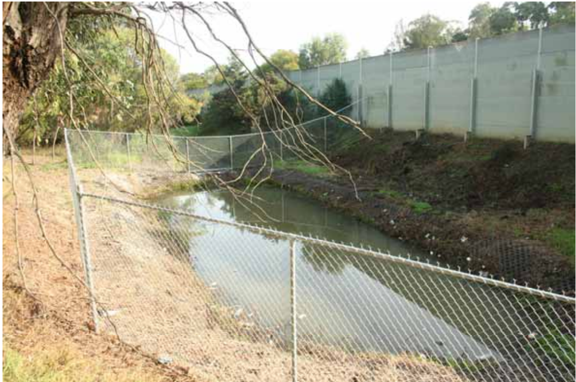
Plate 7: Re-enforced sedimentation basin
