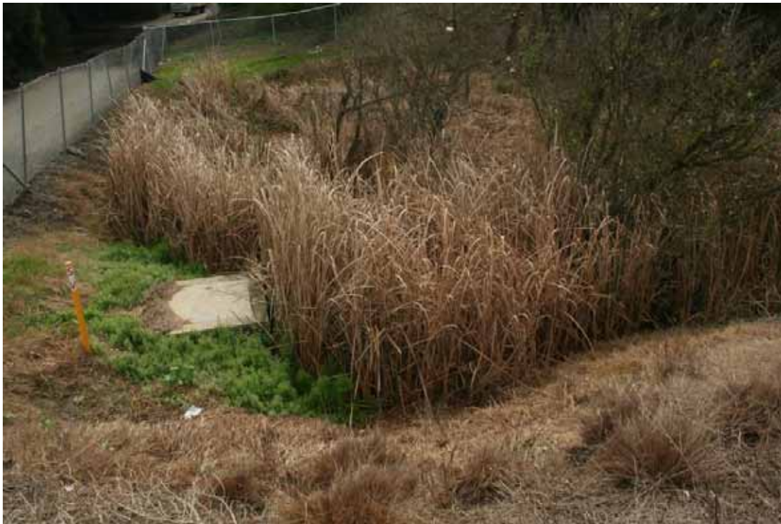
Plate 6: Natural earthen sedimentation basin
