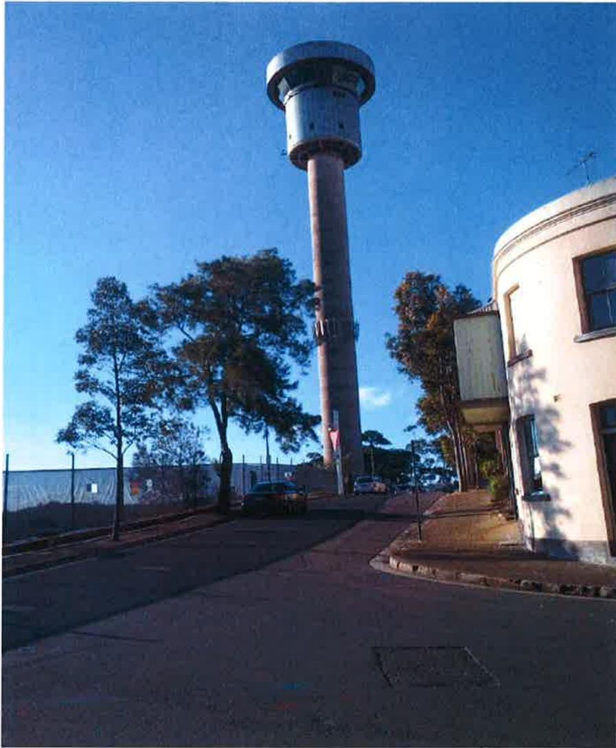
Figure 4: HCT viewed from the corner of Merriman & Bettington streets, Millers Point
