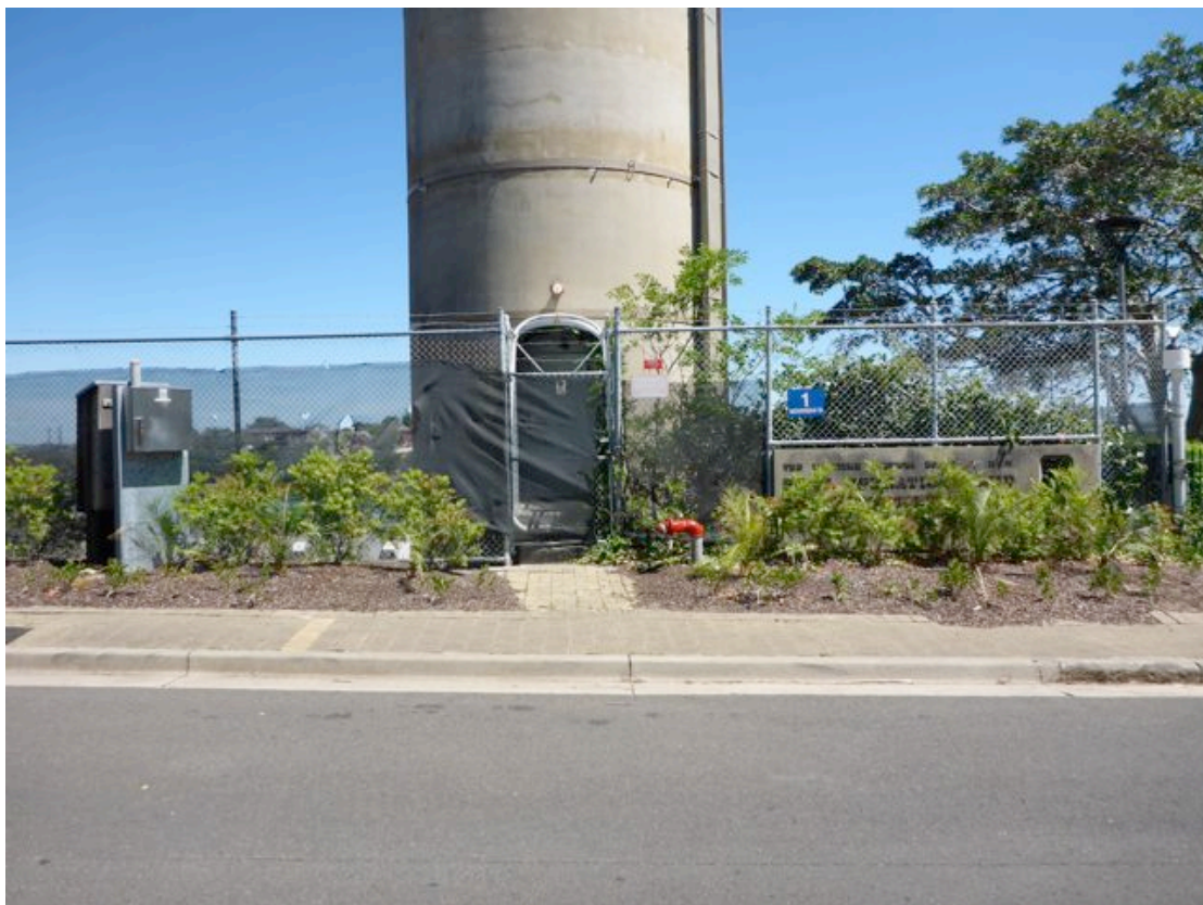
Figure 4.8. Merriman Street entrance to HCT viewed to the west. (Photo Austral Archaeology Pty Ltd, October 2013)
