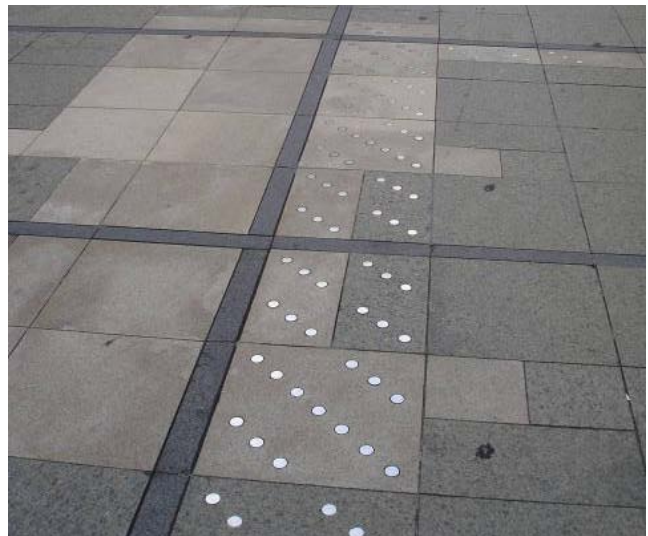
Figure 5.3 Stainless steel 'Dots' and 'inlays' indicating the former walls of Government House at the Museum of Sydney
