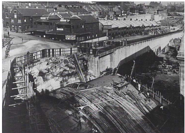
Figure 3.8: Construction of Munn street to Argyle Street.
