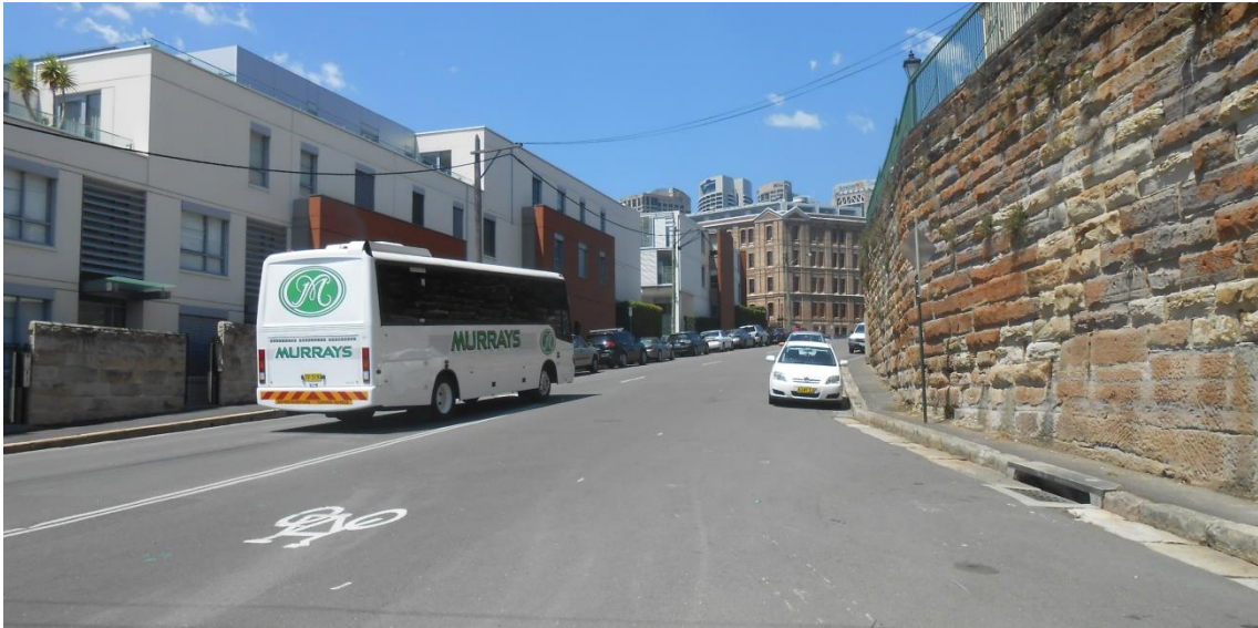
Figure 2.5: Dalgety Road – Mixed Use Cycling Facility
