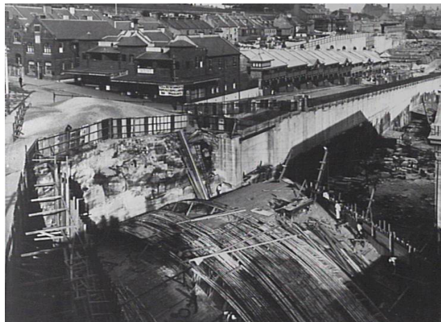
Figure 3.8: Construction of Munn street to Argyle Street.
