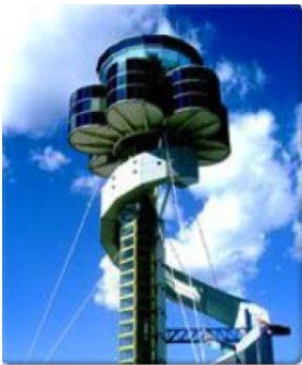
Sydney Airport Control Tower
