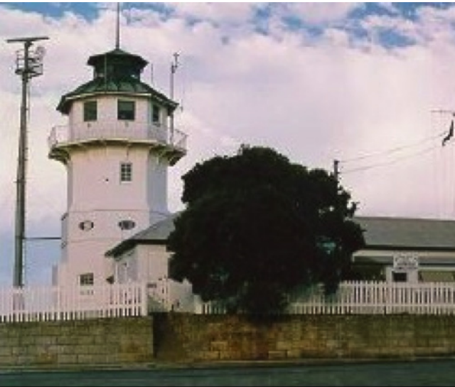
South head Signal Station continued to control shipping into Sydney Harbour until 1992 (Sydney Ports s.170 listing)
