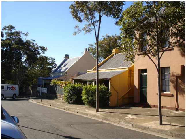
Fig 2.9 Early 1837 housing in Merriman Street opposite the Harbour Control Tower
