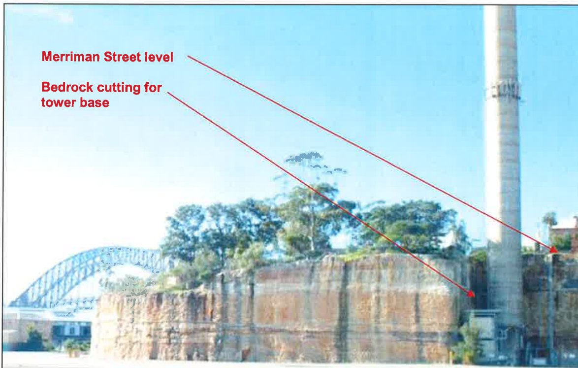
Figure 13: The base of the HCT showing the associated bedrock excavation prior the Headland Park works commencing in 2010. (Source Austral Archaeology)
