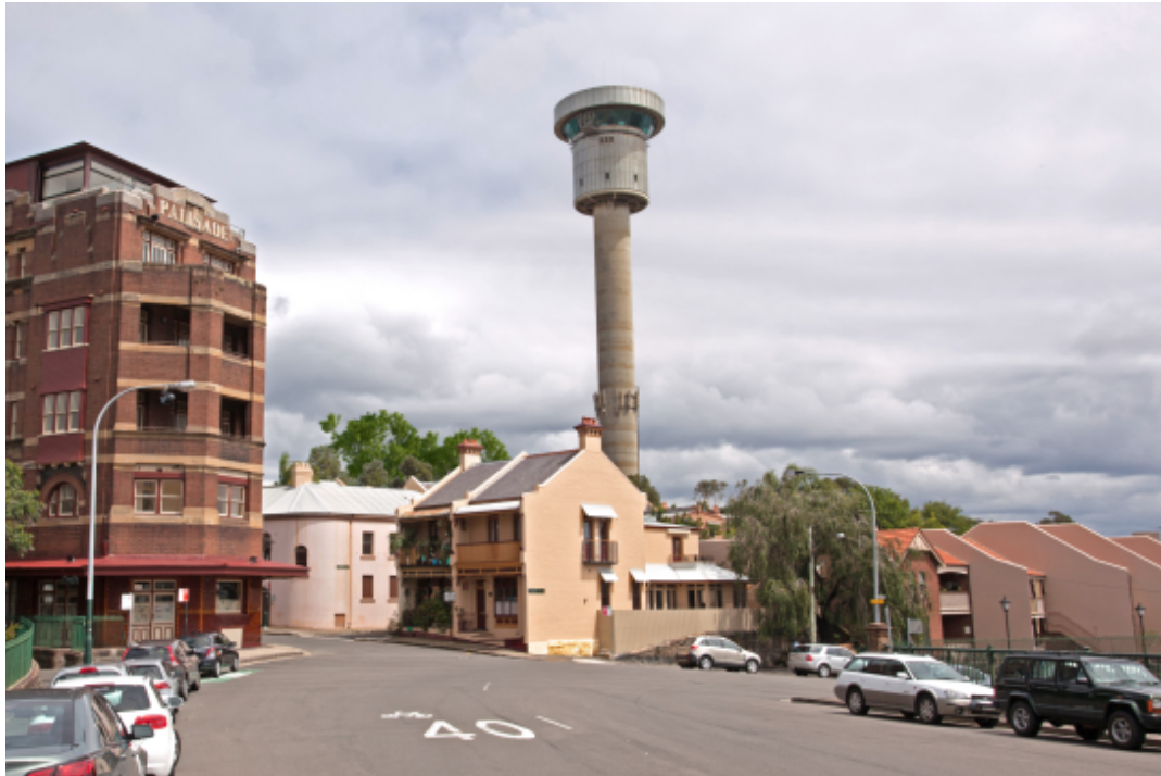
Photomontage P3 - Argyle Street toward Dalgety Road intersection, existing view
