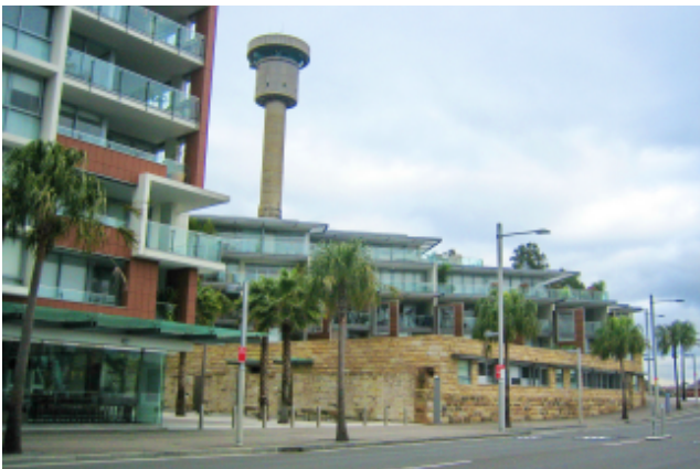
Photo Location 3 - Towns Place (toward future Headland Park)
