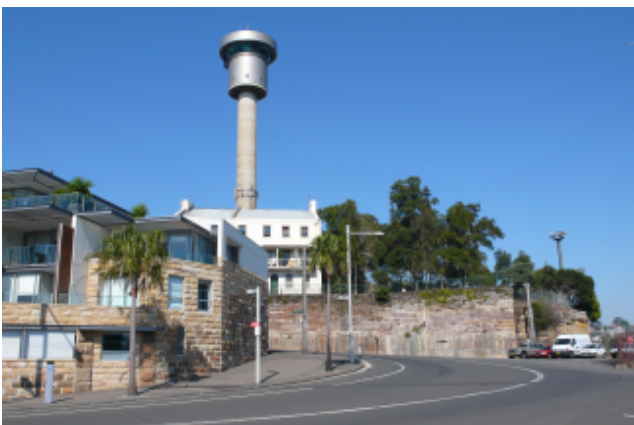
Photo Location 5 - Towns Place (toward Dalgety Road)
