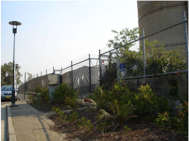
Fig 2.2 View of HCT and fence to Merriman Street.
