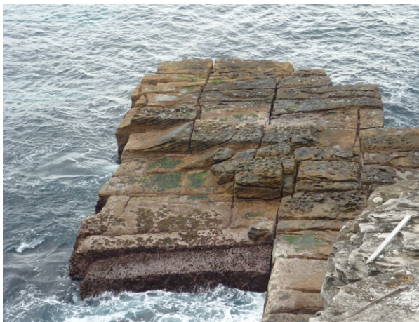
Naturalistic rock platforms constructed from geometric forms
