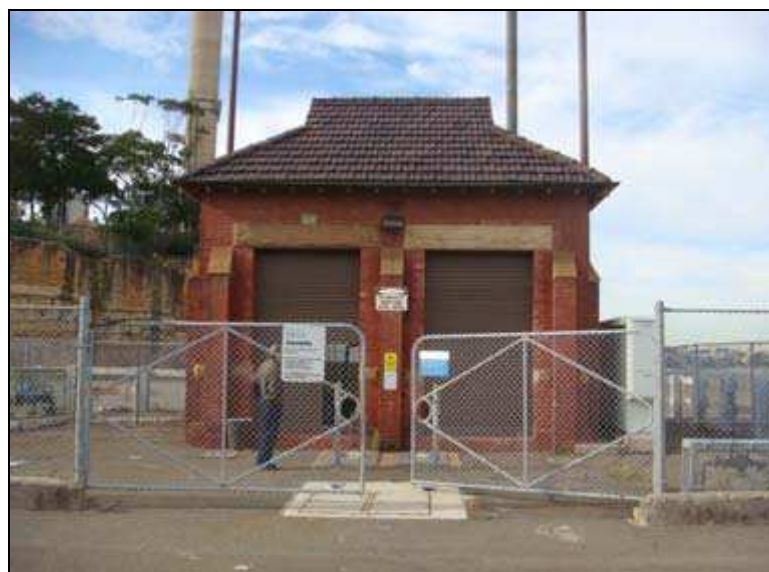
Figure 15: Sewage pumping station
