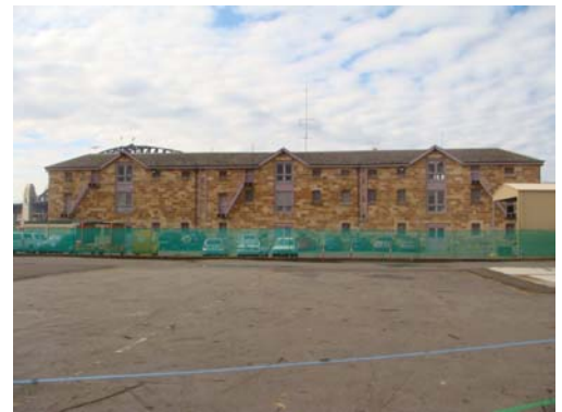
Fig. 3.14: Moores Wharf Building viewed from west.
