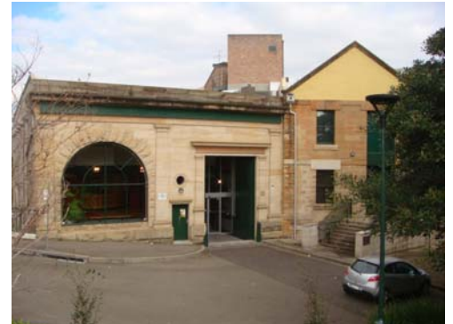
Fig. 3.6: Dalgety's Bond Store from Munn Street Reserve.
