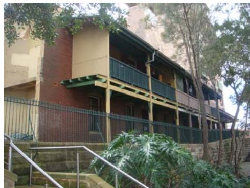
Fig. 3.7: View of 18-20 Munn Street Terraces from south-west.
