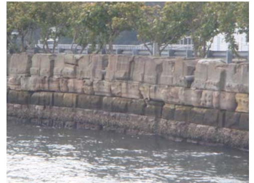
Fig. 3.4: Sandstone seawall with stormwater pipes penetrating through.
