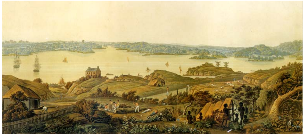
Fig. 2.6: c1821 image of the Inner Harbour looking west from Flagstaff Hill (Observatory Hill). Millers Point is the peninsular with John Leighton's windmills. Note the depiction of the relatively steep cliffs and knolls on the southern side of Millers Point.
