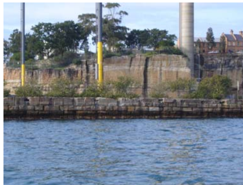
Fig 3.3: View of sandstone seawall at north-west corner of site.
