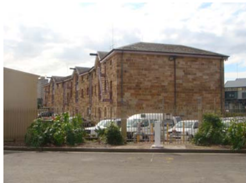
Fig. 3.13: Moores Wharf Building viewed from south.
