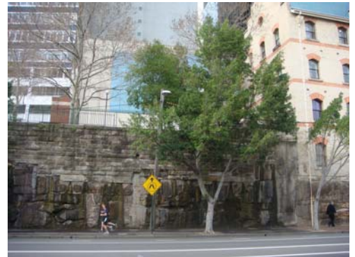
Fig. 3.10: Sandstone wall adjacent to Grafton Bond Stores.
