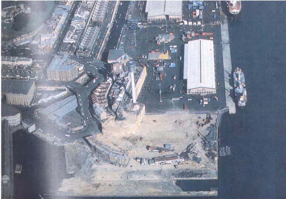
View to the south demonstrating the reconstruction of the headland 1970s. Moore's Wharf is in its original position and the shape of the original headland can be partly discerned by the location of the remaining buildings. The existing sandstone sea wall can be seen on the western side of the headland and the concrete sea wall constructed in 1904 is evident behind the concrete caisson at the bottom of the image. (Source: Maritime Services Board Annual Report 1977-78, p 8)
