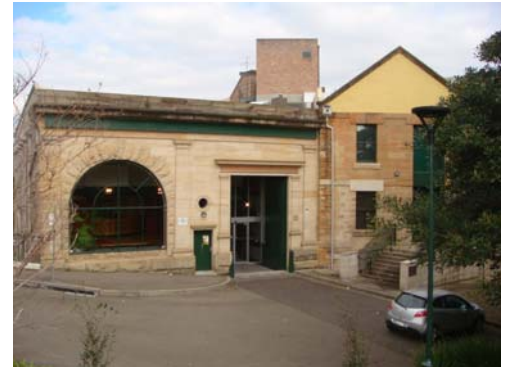
Fig. 3.6: Dalgety's Bond Store from Munn Street Reserve.
