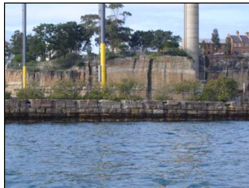
Fig 3.3: View of sandstone seawall at north-west corner of site.
