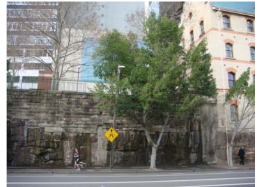
Fig. 3.10: Sandstone wall adjacent to Grafton Bond Stores.
