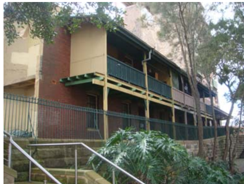
Fig. 3.7: View of 18-20 Munn Street Terraces from south-west.
