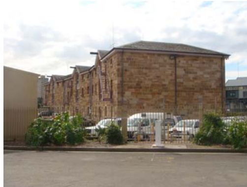
Fig. 3.13: Moores Wharf Building viewed from south.
