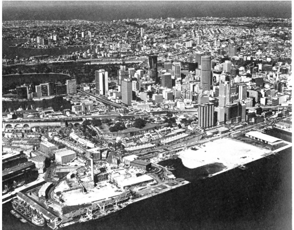
Fig. 2.16: 1971 image of Millers Point indicating the reclamation of the site for containerization, the construction of the Harbour Control Tower and the further cutting away of sandstone for the creation of flat dock area
