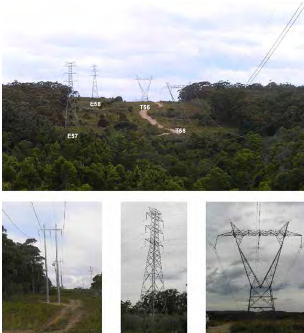
Figure 34: Power transmission lines above Longwalls 1 and 2.
