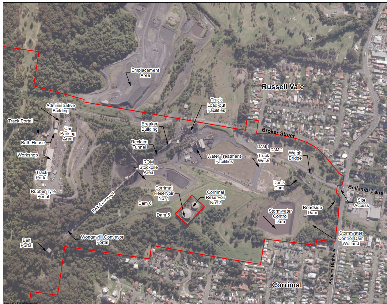
Figure 4 – Surface Facilities Site
