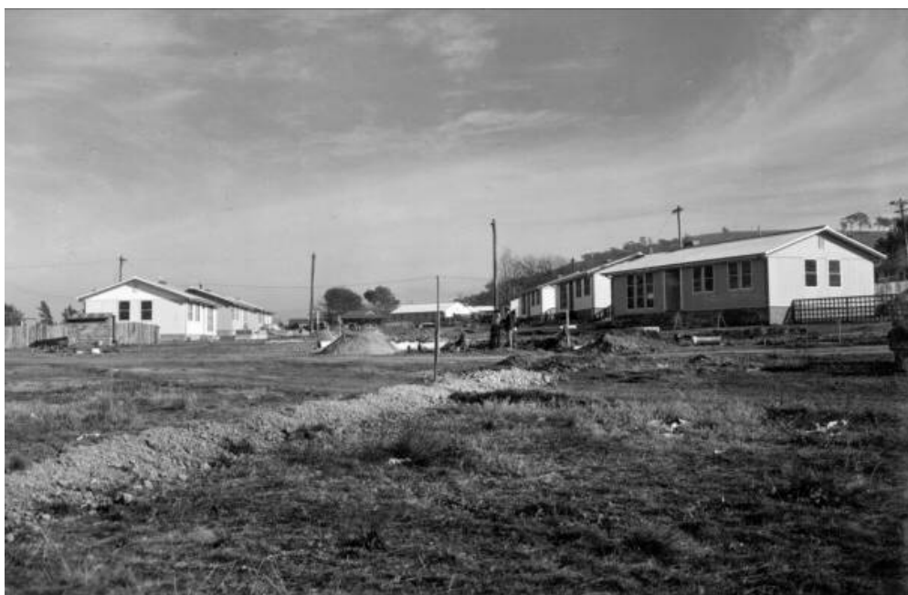
Figure 4.8 Typical examples of Riley-Newsum pre-fabricated type government housing, under construction at Duntroon, 1951 (AHC 001314).
