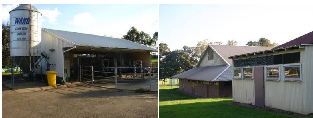
Figure 5.4 The dairy (left) and associated farm buildings (right).
