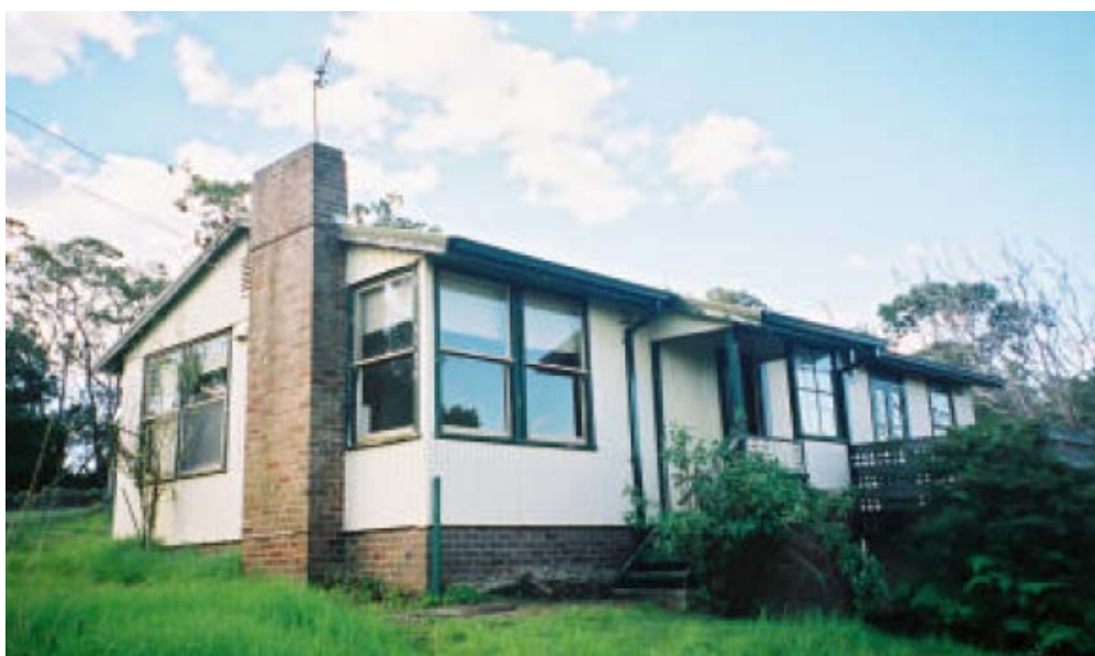
Figure 4.9 Amals Sagverks Aktiebolag prefabricated cottage, 7 Commonwealth Ave, Georges Heights (Robertson & Hindmarsh 2004).
