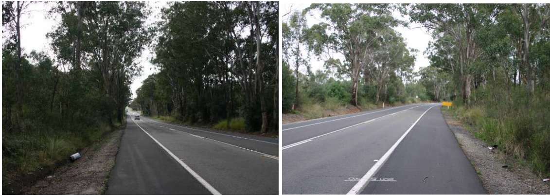
Figure 5.16 View to the east and the location for the bridge, and west along Campbelltown Road.
