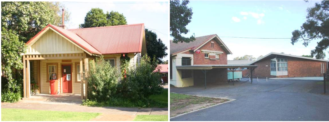
Figure 5.5 The prefects' cottage (left) and the juxtaposition of 1920s and 1960s buildings (right).
