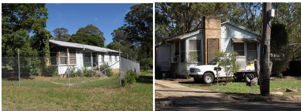
Figure 5.21 The Amals Sagverks Aktiebolag cottage at 8/10 Flinders Crescent (left), and the cottage at 7 Blaxland Rd.
