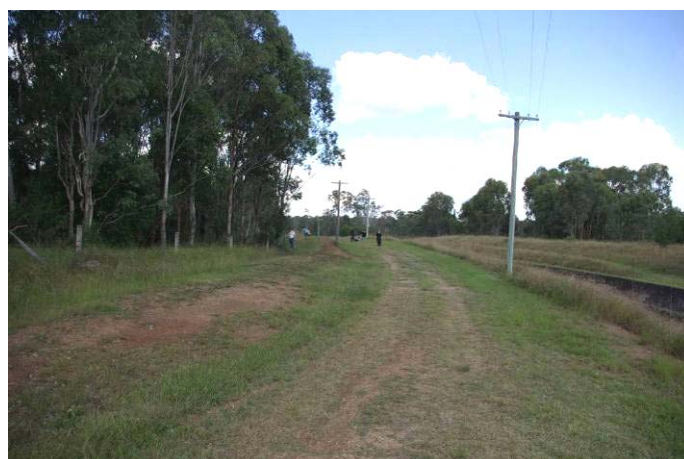
Figure 5.26 View south to SWRL Site 7, showing Canal (right) and SCA boundary fenceline (left).
