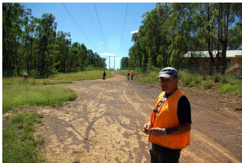
Figure 5.36 View north east of SWRL Site 10.
