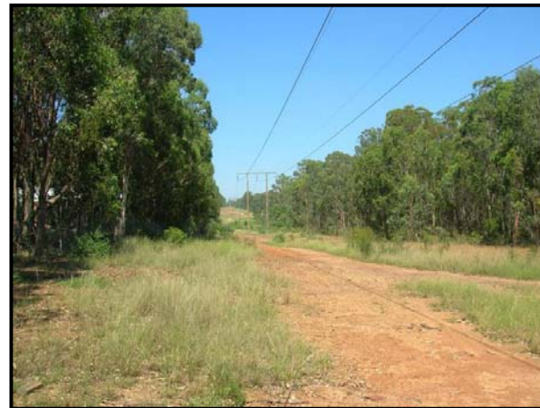
Figure 2.5: Transmission line cuts through Denham Court residential area and area of Shale Hills Woodland.
