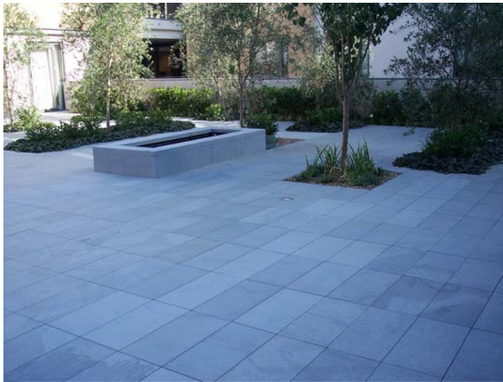
STACKBOND GRANITE PAVING
