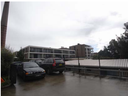
Figure 13: Modern Flat Building, 88-98 King Street. This is the immediate context of the development to the west.
