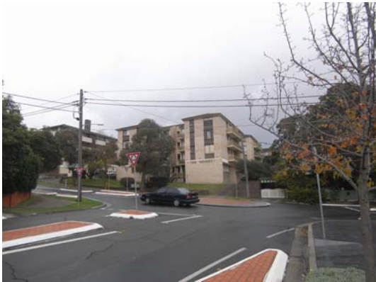
Figure 11: Modern flat building, 113-123 King Street. This is the immediate context of the development to the south-east.
