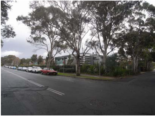
Figure 9: View to the site of proposed buildings on the horizon from corner of Dangar Street and Govett Lane.
