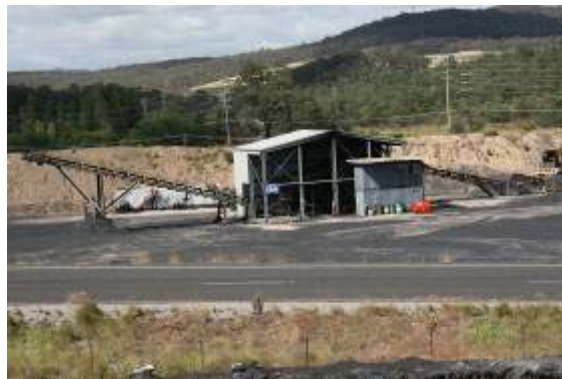
Plate 1.3 Crushing, Stockpiling and Maintenance Area
