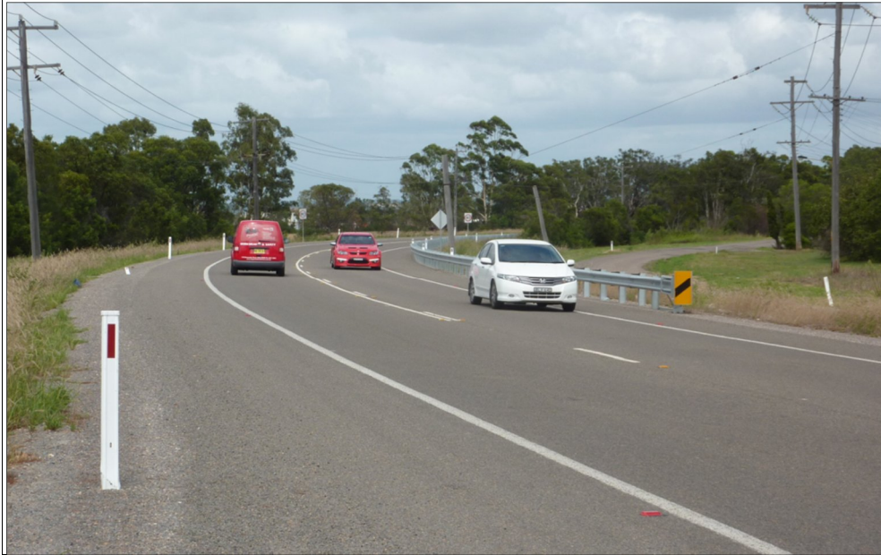
Figure 4 Tomago Road (looking west towards approach to McIntyre Road)
