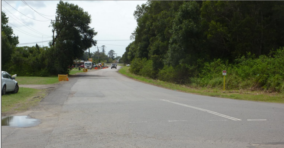
Figure 6 School Drive, view looking east towards turnoff to Tomago Road
