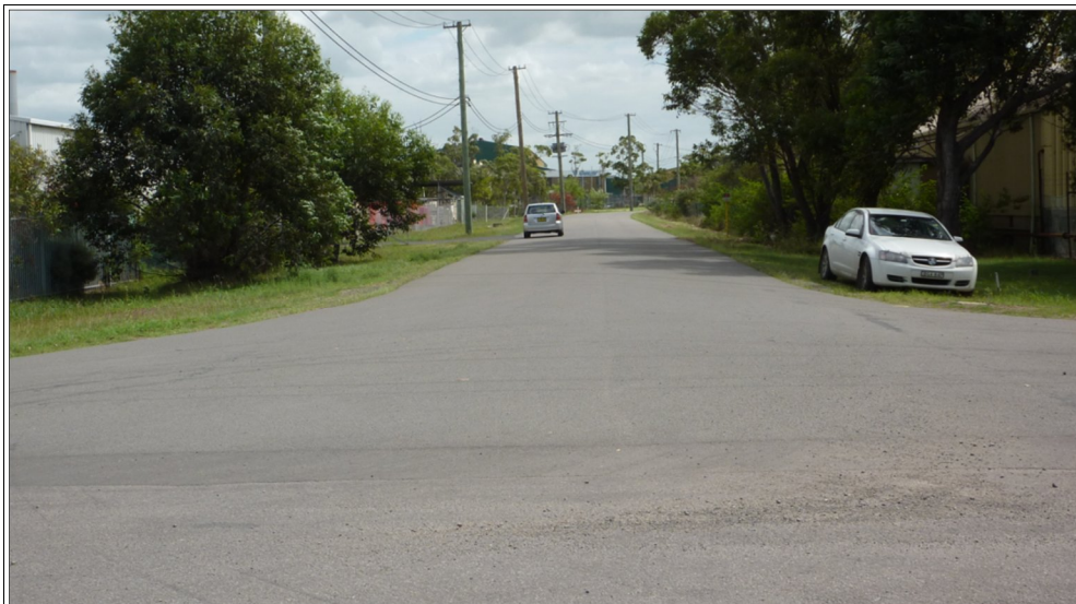
Figure 7 Private Road looking north from School Drive
